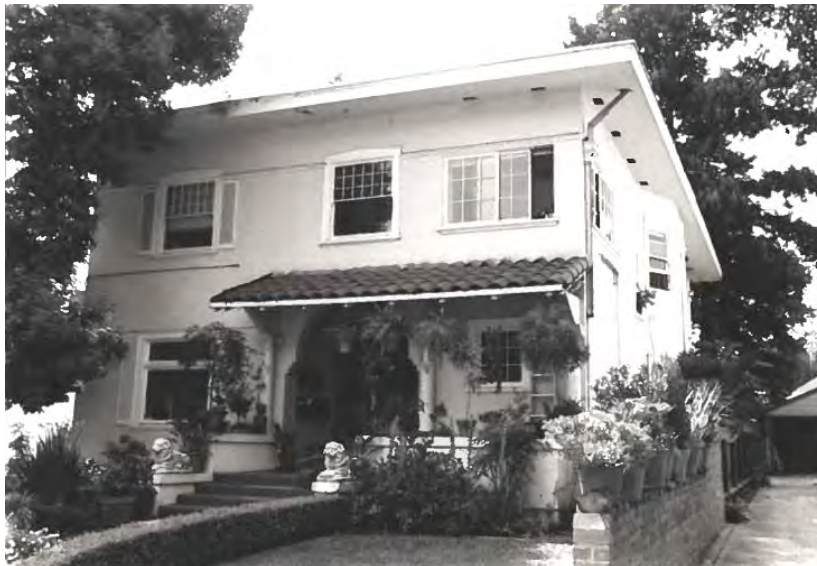
Figure 1: 1997-2001 Survey Update photograph of 818-820 Cowper Street.
