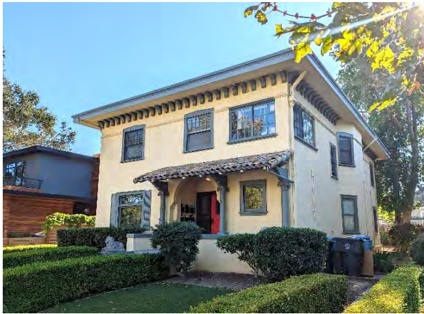
Figure 2: 828-830 Cowper Street, 2023 Reconnaissance Survey photograph.
