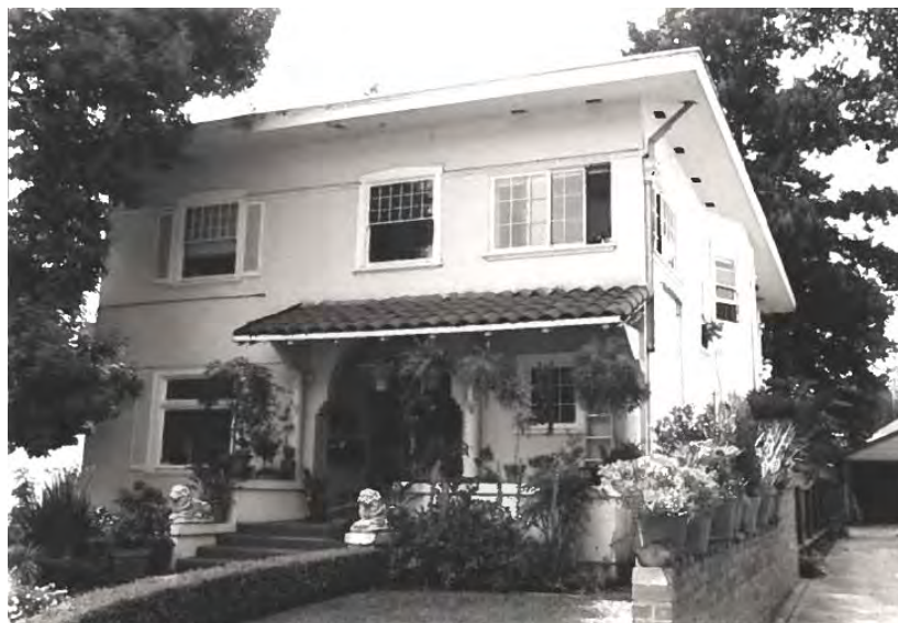
Figure 1: 1997-2001 Survey Update photograph of 818-820 Cowper Street.
