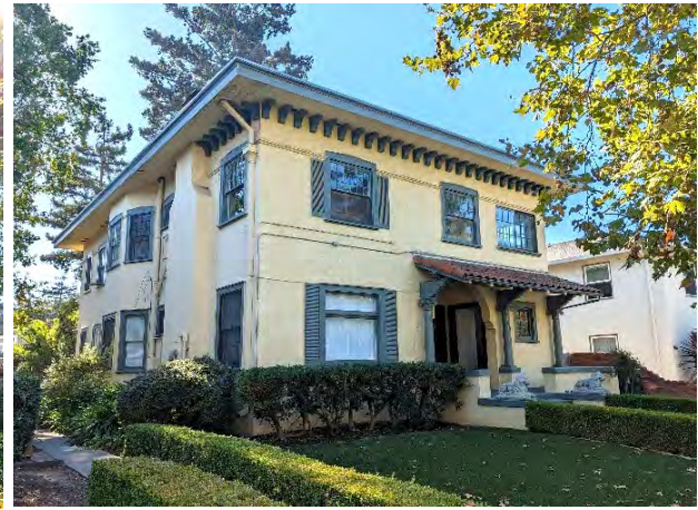
Figure 3: 818-820 Cowper Street, 2023 Reconnaissance Survey photograph.
