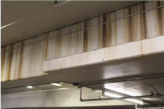
Civic Center Parking Garage, February 2015
