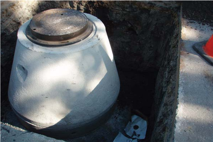
Sewer manhole base
