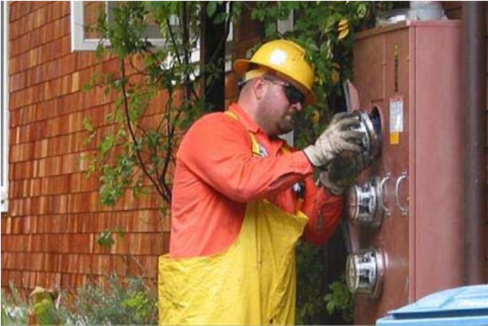
Electric Troublemaker installing an electric meter to provide service to a customer
