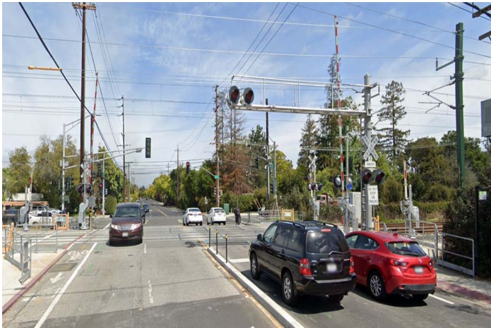
Caltrain Crossing at Meadow Drive, January 2023
