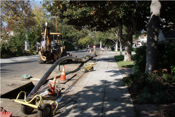
Installation of 8" HDPE pipe by directional drilling method
