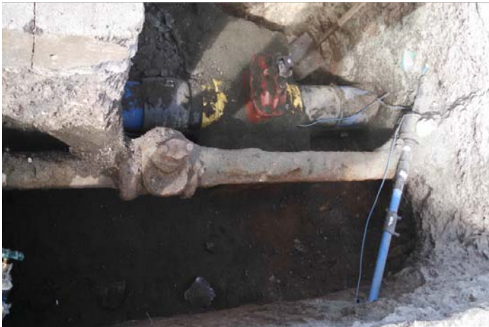
Old Water Main being Replaced
