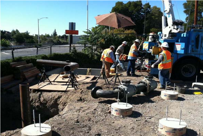
Installation of new HDPE gas service main
