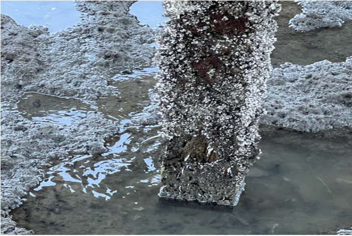
Boardwalk piling decay
