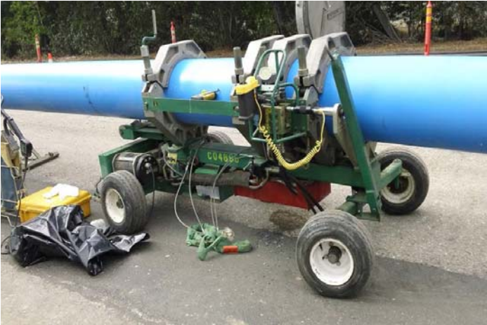
16" HDPE pipe being fused prior to installation
