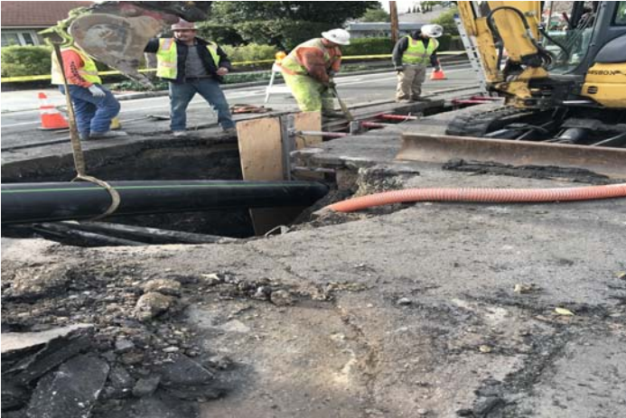
Construction crew installing wastewater main
