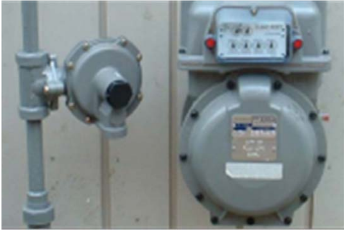
New gas service meter and regulating equipment
