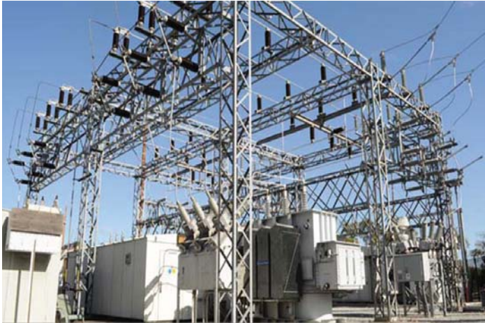
Electric Substation transformer and bus structure
