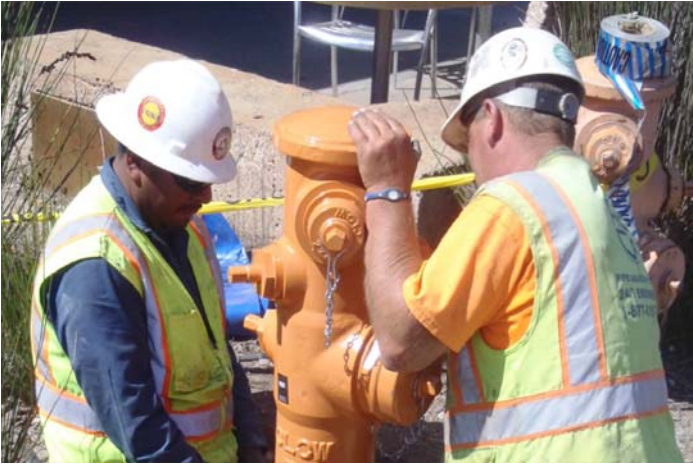
Installation of a new fire hydrant with FlowGuard fire hydrant check valve
