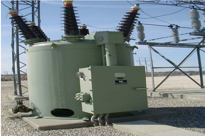
High voltage circuit breakers
