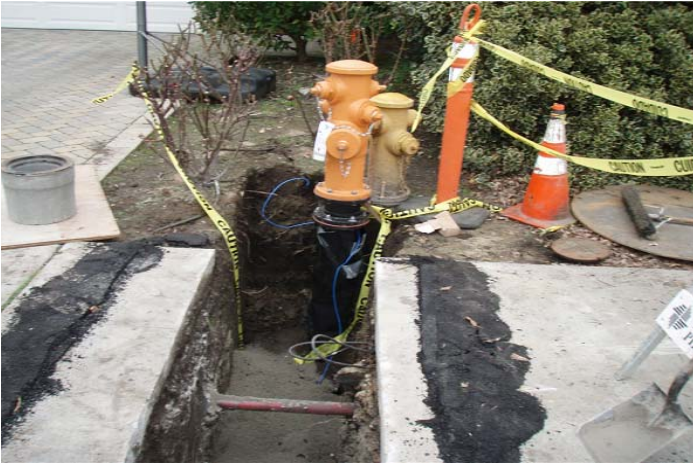
Newly installed fire hydrant service line and assembly on Greenwood Avenue
