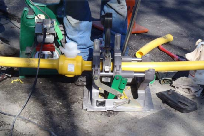
New HDPE gas pipe being fused prior to installation
