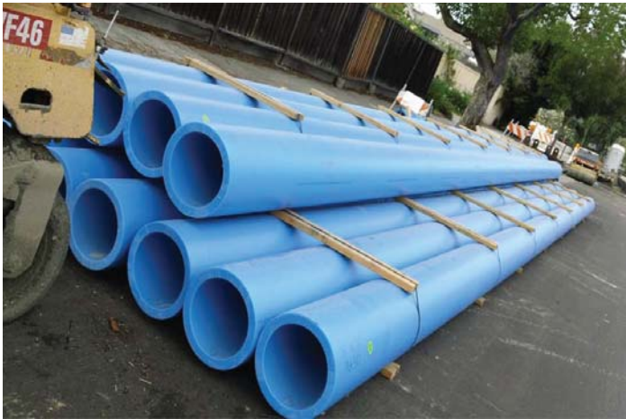
HDPE pipe waiting to be fused
