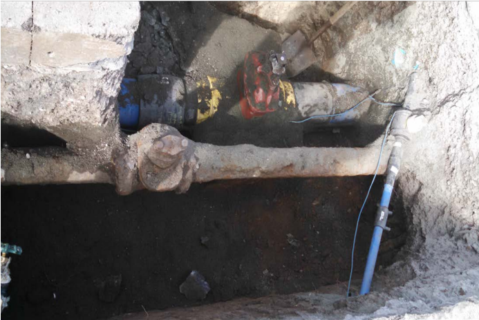
Old Water Main being Replaced
