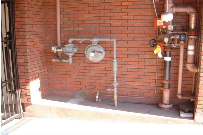
New gas service meter and regulating equipment
