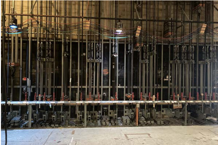
Fly rail of the rigging system at the Lucie Stern Community Theatre
