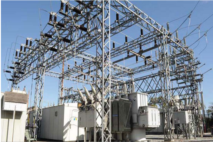
Electric Substation transformer and bus structure
