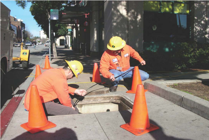
Fiber optic crew installing new fiber optic cables
