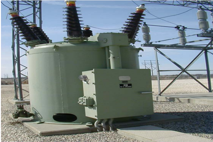
High voltage circuit breakers
