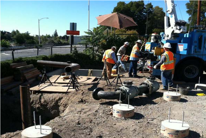
Installation of new HDPE gas service main
