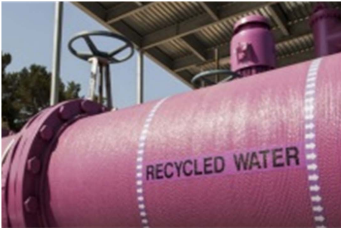
Recycled water piping
