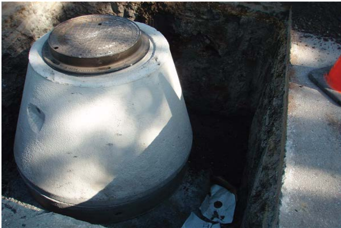
Sewer manhole base
