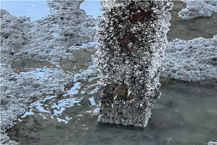
Boardwalk piling decay
