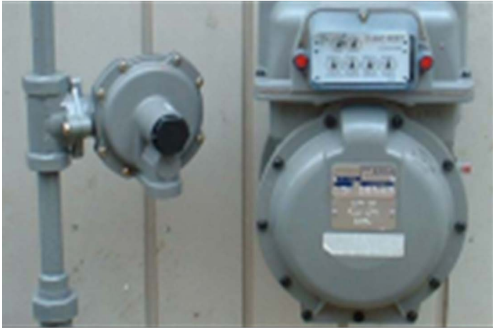
New gas service meter and regulating equipment
