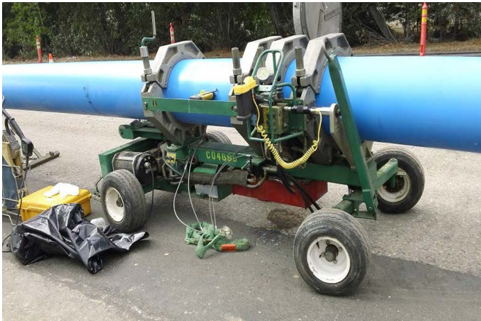
16" HDPE pipe being fused prior to installation
