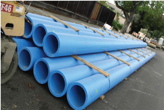
HDPE pipe waiting to be fused
