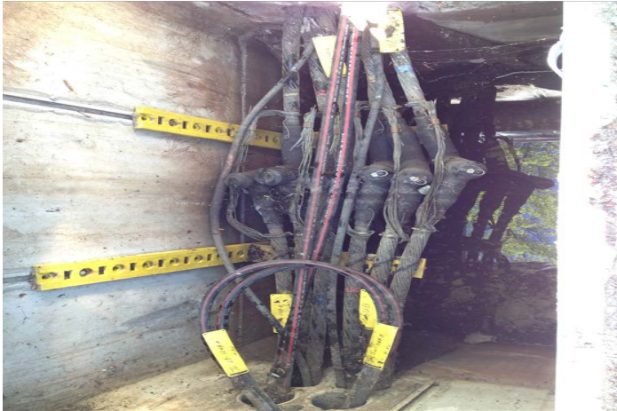
Electric underground cable vault
