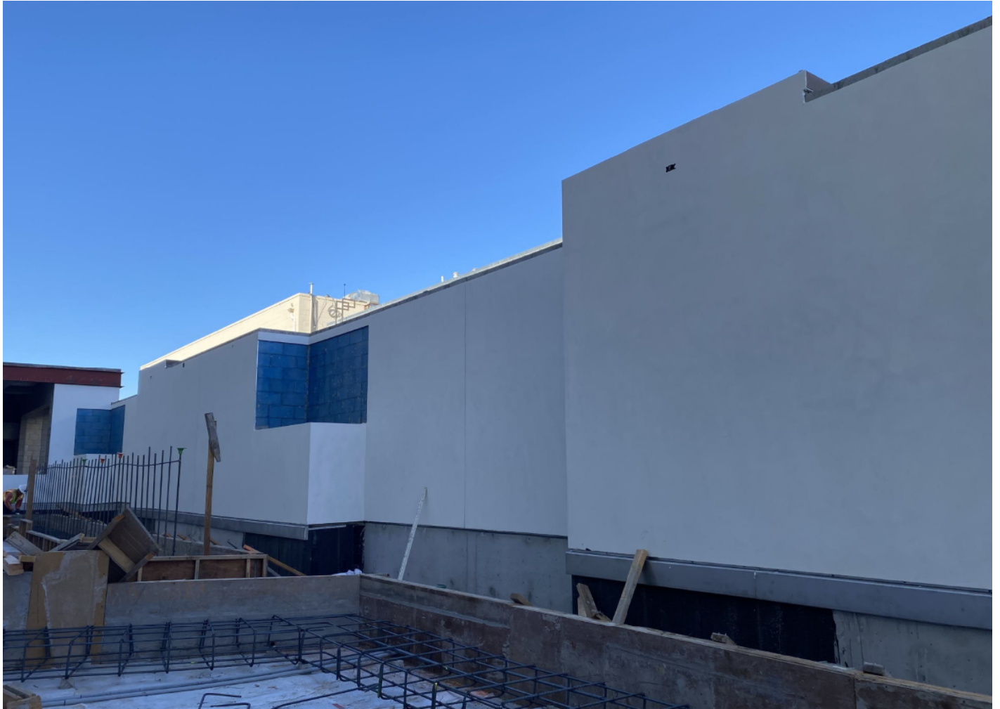
View of Jacaranda Plaster Walls.
