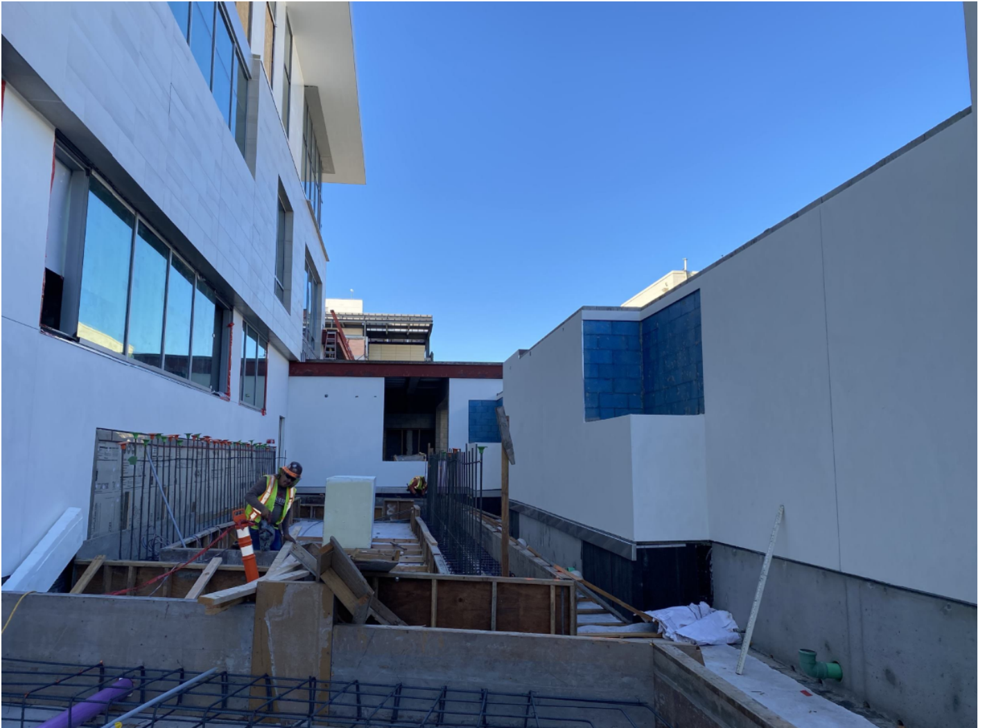
View of CMU plaster and site work on Jacaranda Rd.
