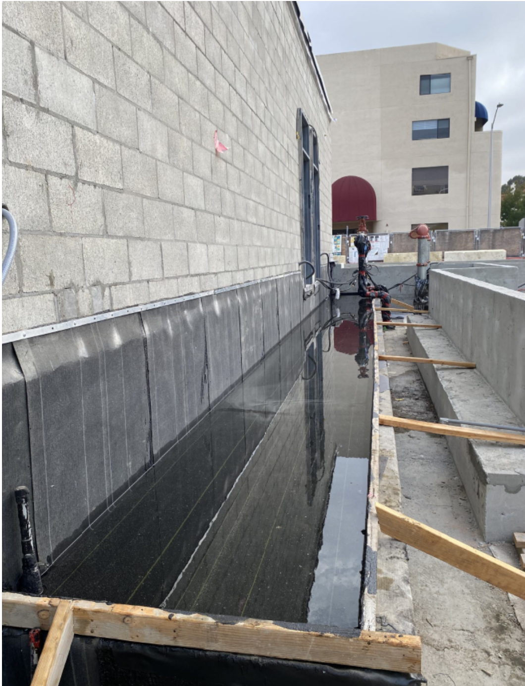
Waterproof flood testing.
