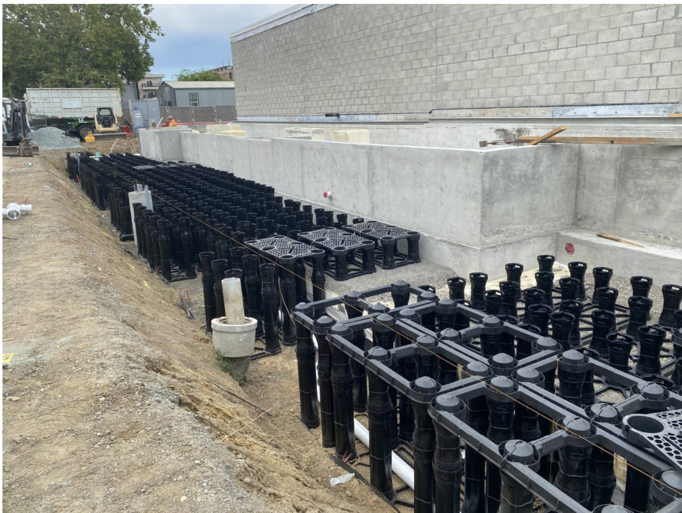
Silva Cell installation on Park Ave.
