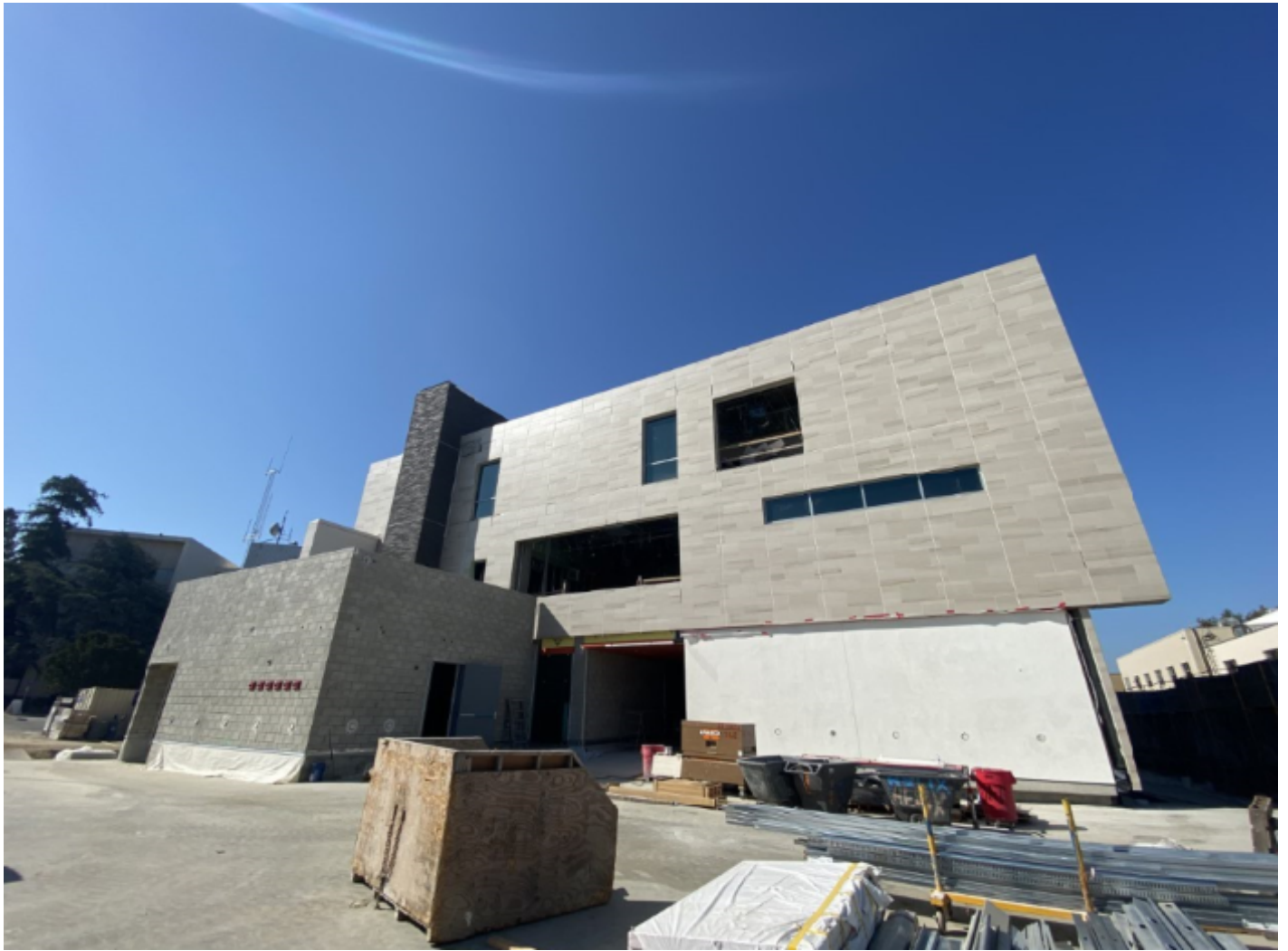
View of building East elevation from Utility Yard.
