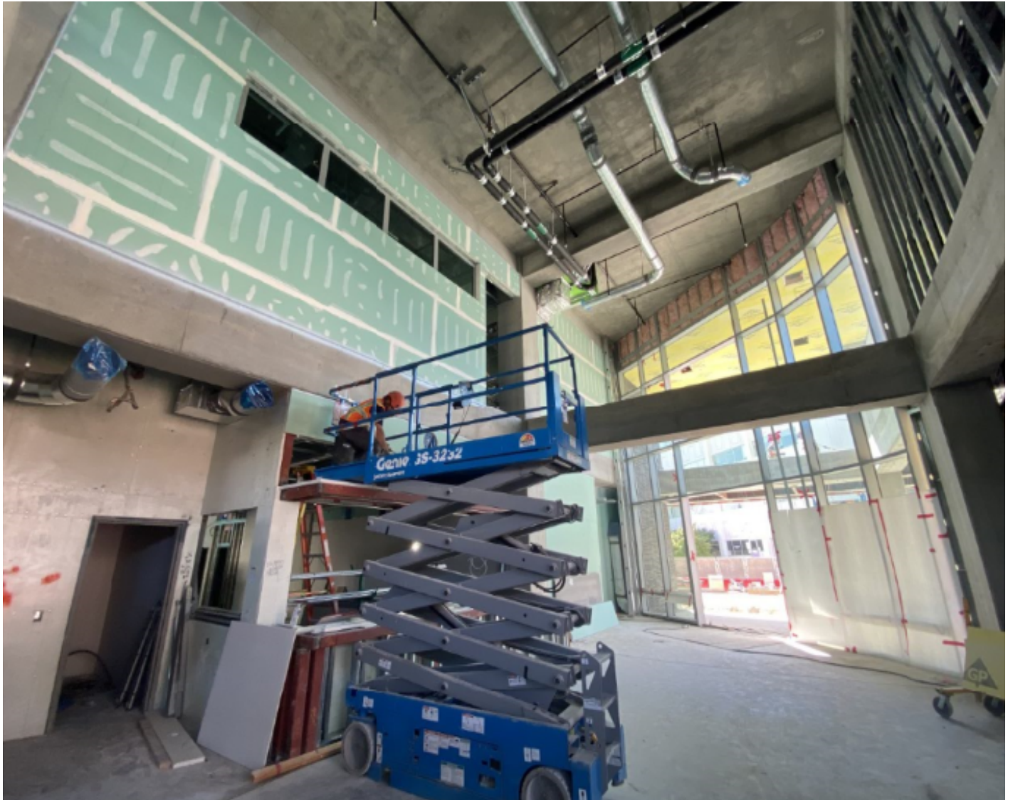
Ongoing work in public lobby area.
