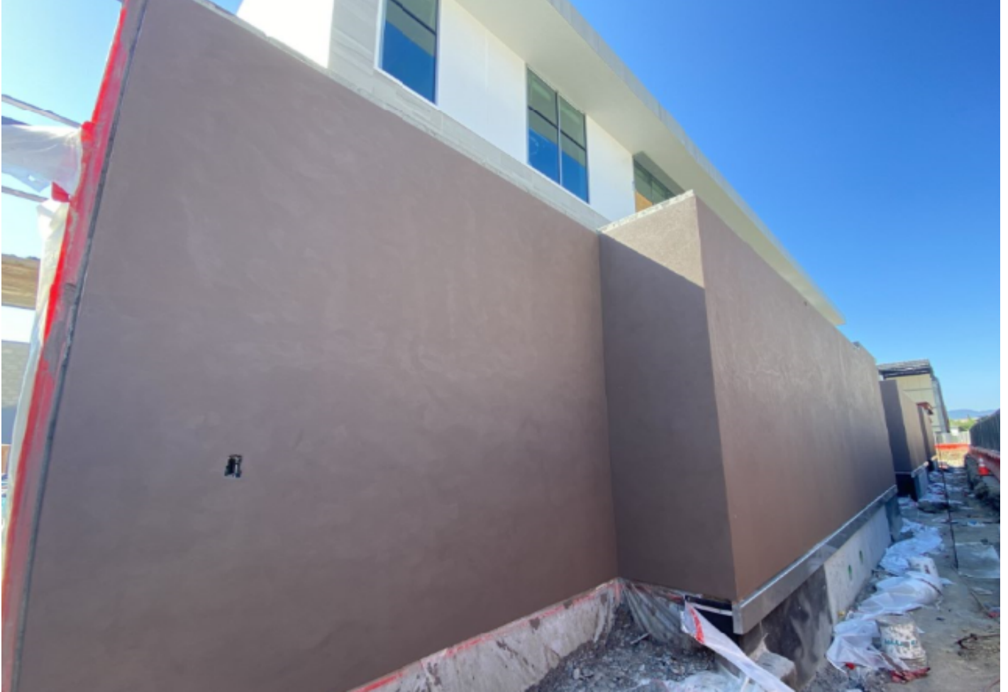
View of CMU plaster on Jacaranda Rd.
