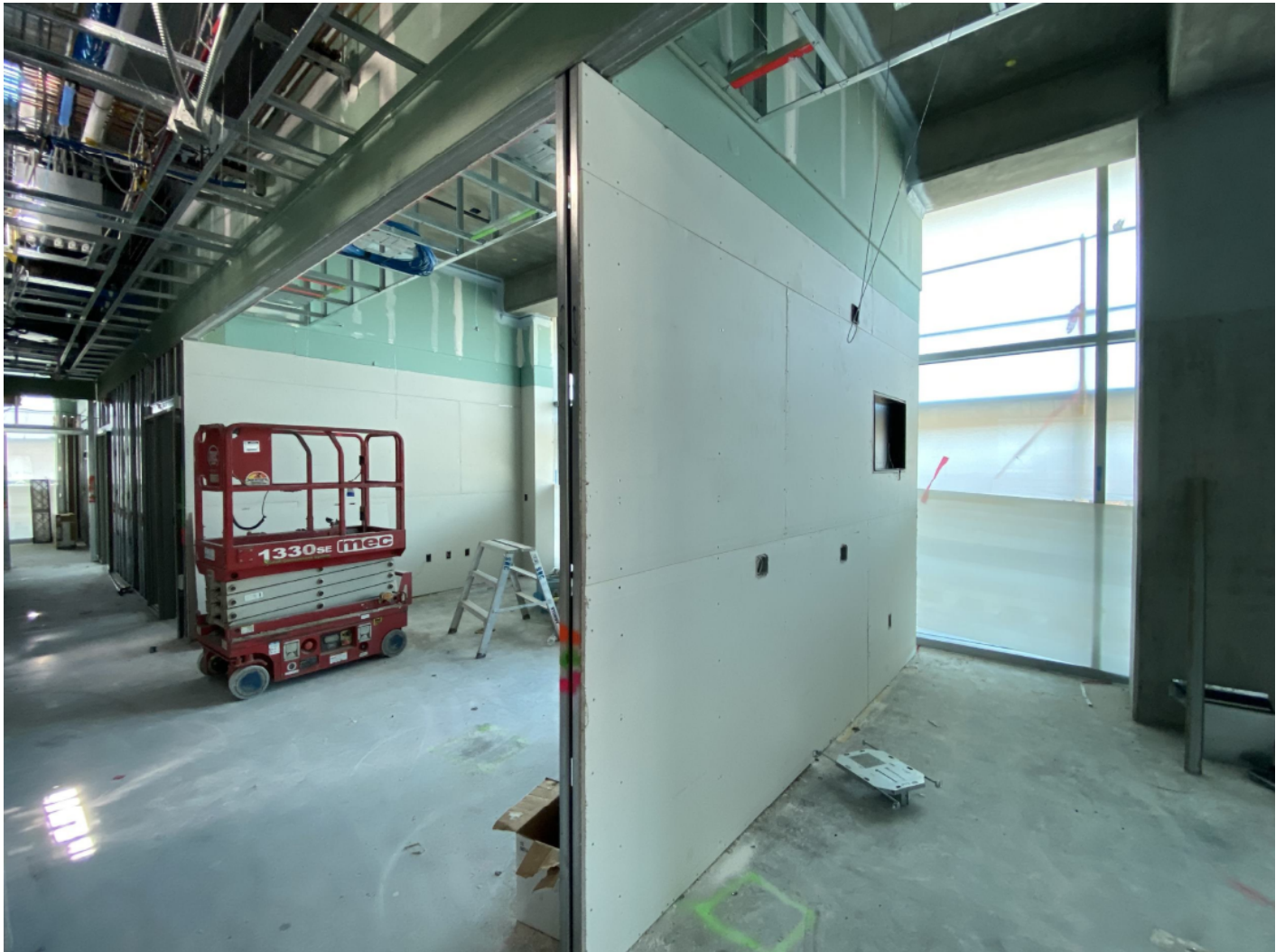
Single side drywall Level 3.
