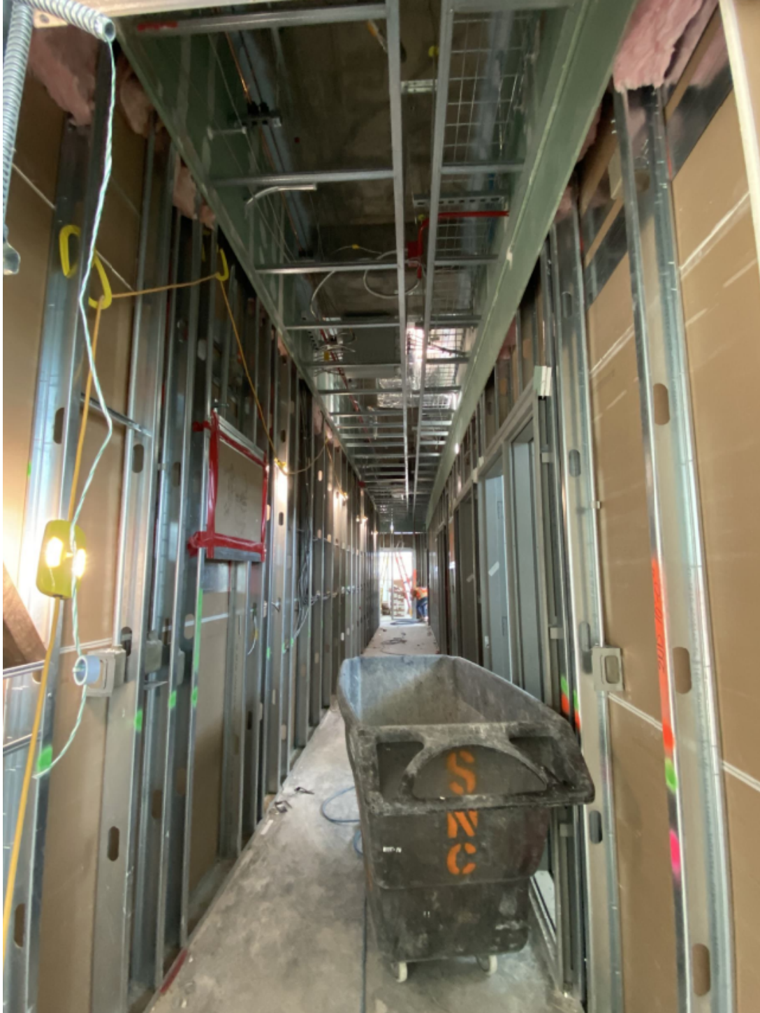
Single side drywall Level 3.
