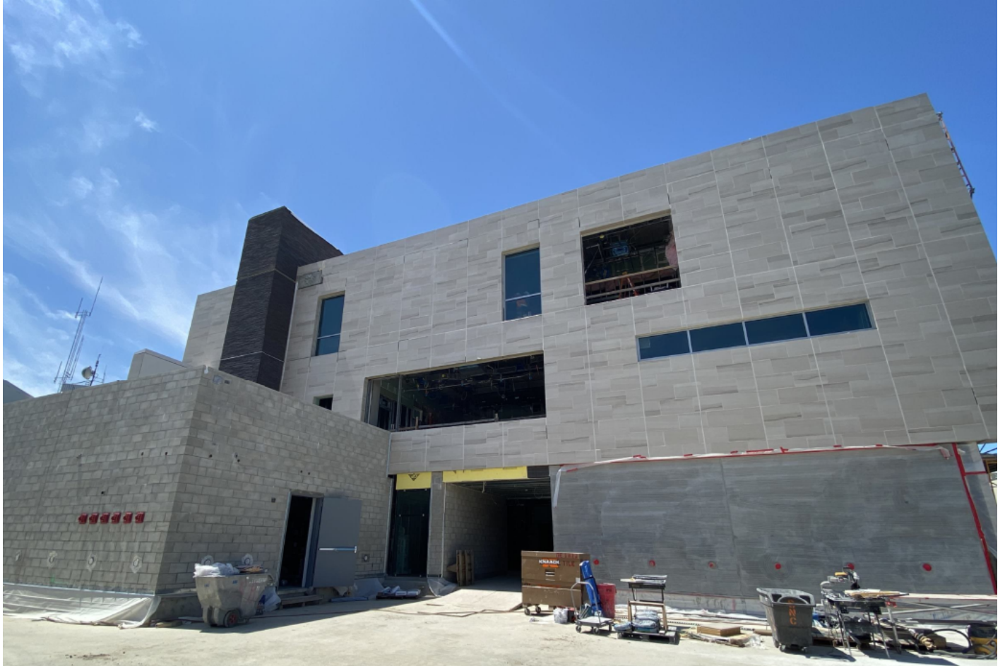
View from Utility Yard looking at East Elevation of the Building.
