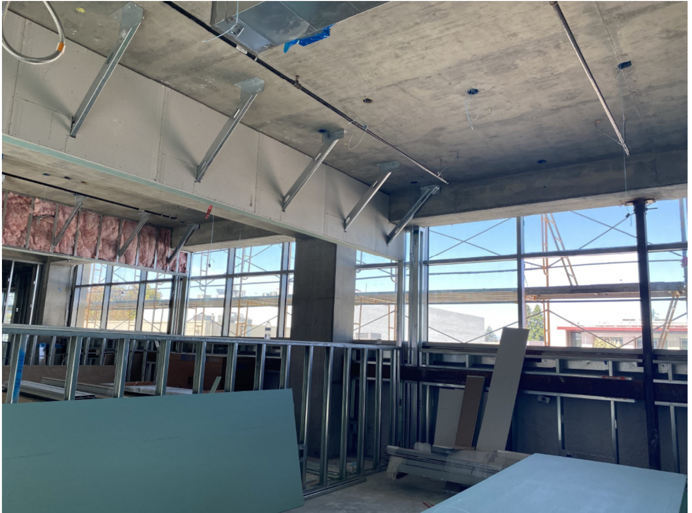
Wall header kickers on Level 2.
