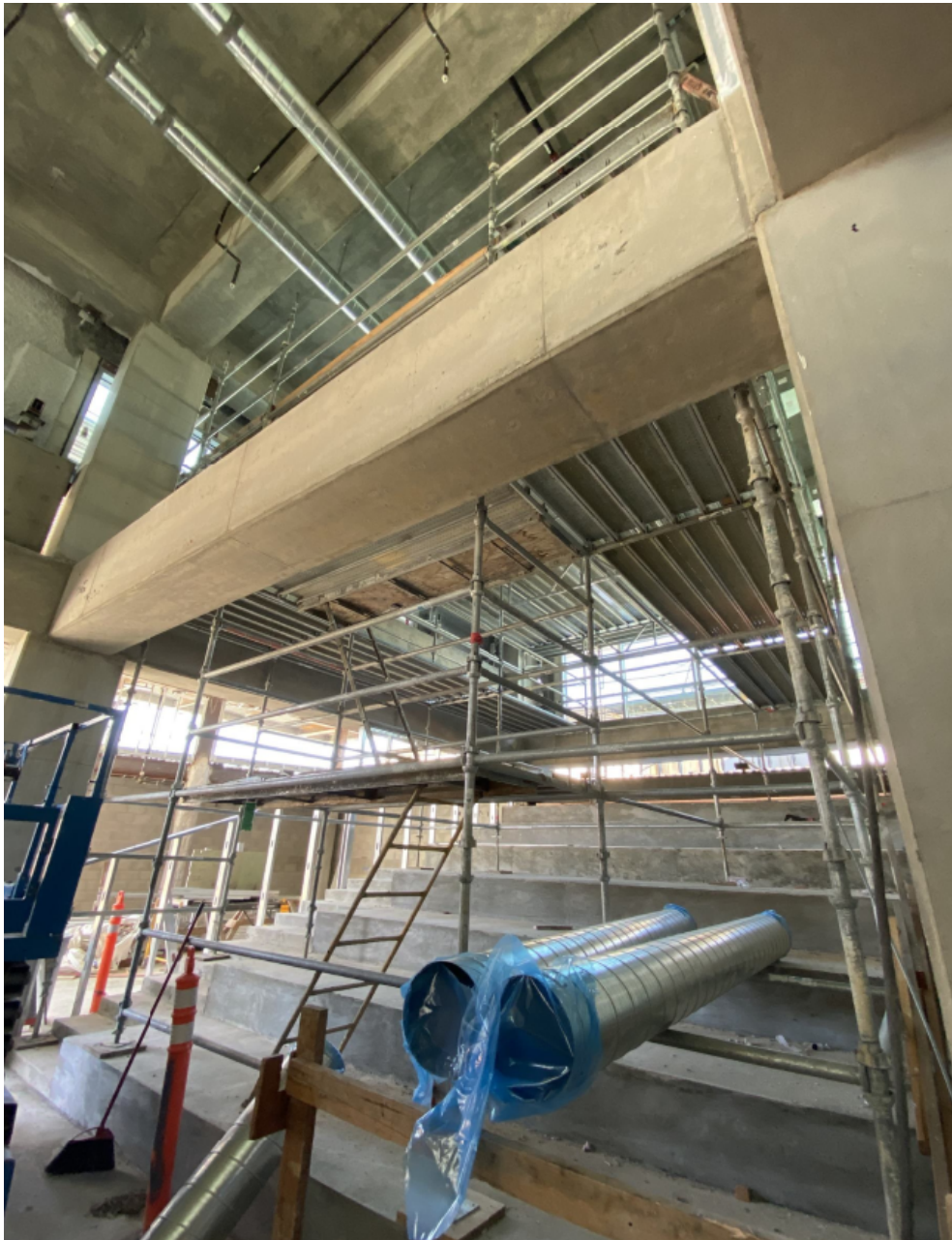
Scaffold at Lobby seating area.
