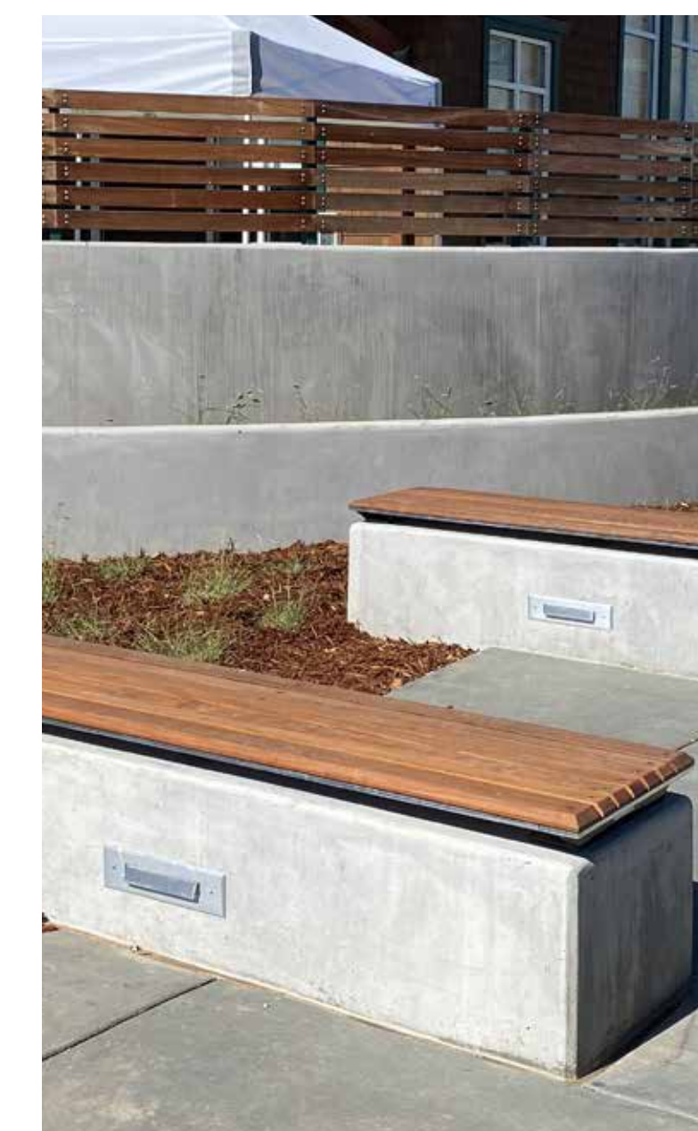
Cast in place seatwall with wood bench top
