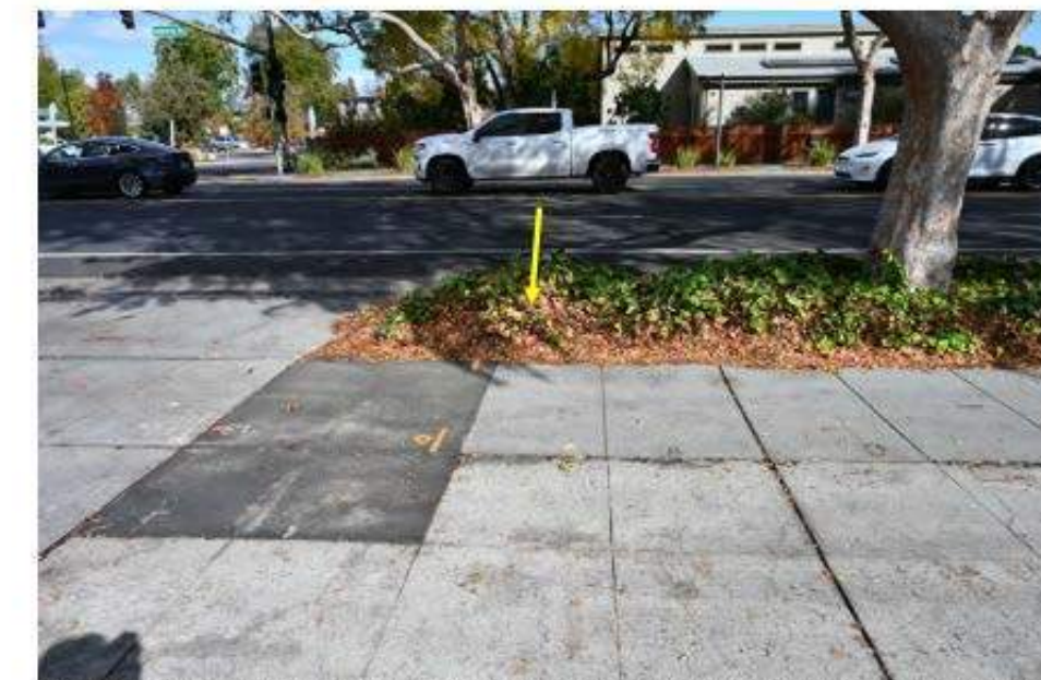
The area where the planter will be reduced to allow for widening of the driveway (see site plan). Note sidewalk repair that likely removed roots causing displacement.
