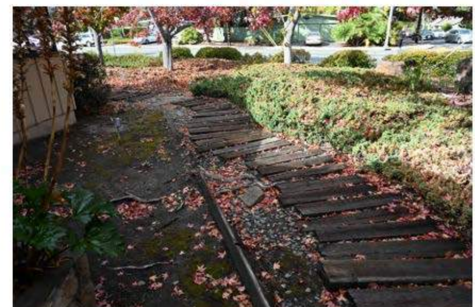
Surface roots extend 30 feet from the base of the tree. This area will be excavated for the new building foundation.
