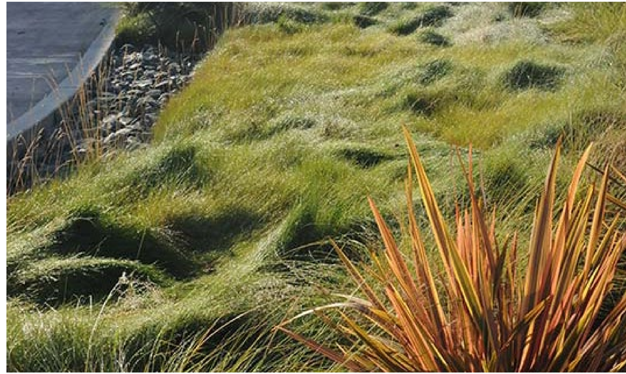
Bioretention with biofiltration sod
