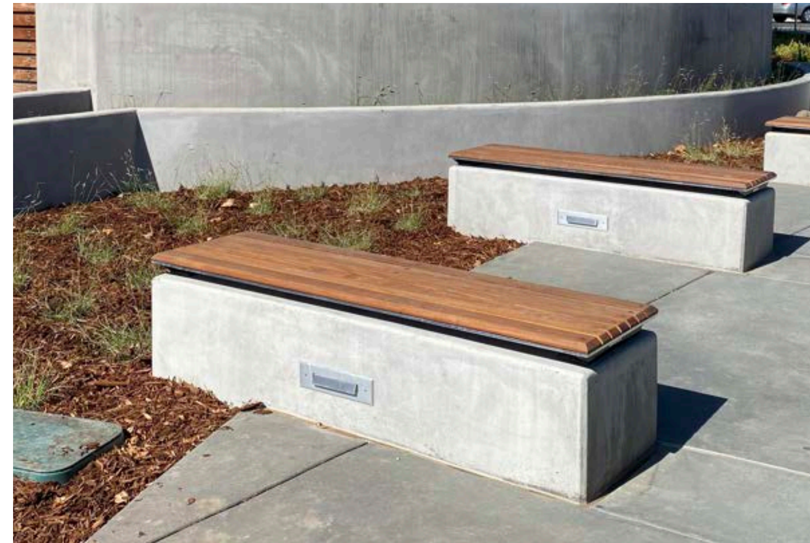
Cast in place seatwall with wood bench topper
