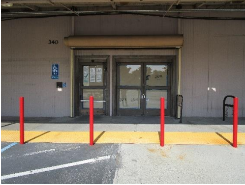
Fenestration (wood frame windows; garage door openings; wire glass skylights over former warehouses)
