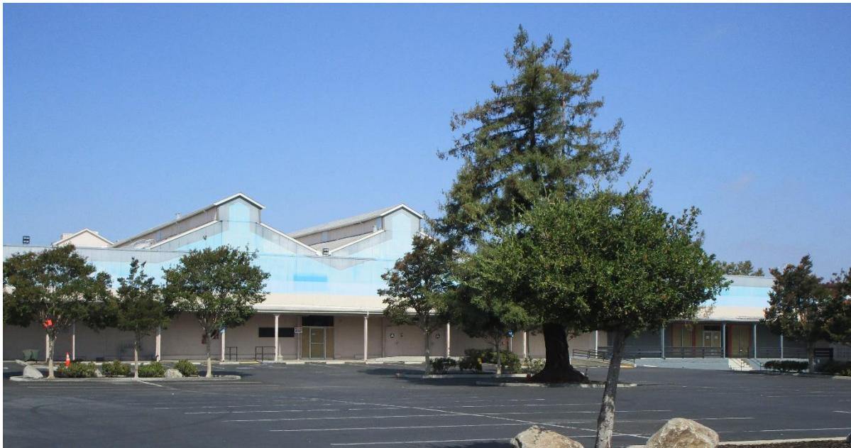
Figure 9 South Elevation of the former canning/warehouse building at 340 Portage Avenue
