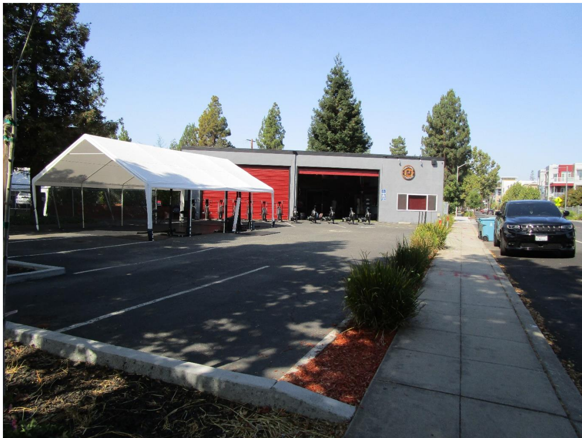
Figure 8 South Elevation of 3040 Park Boulevard, View North
