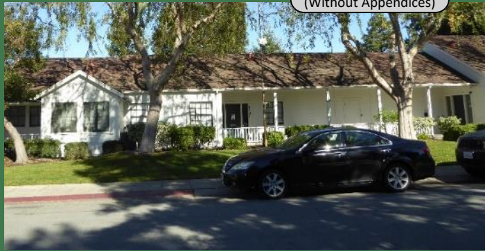
Figure 13 A portion of the southwest facade of the former office building. Source: Page & Turnbull
