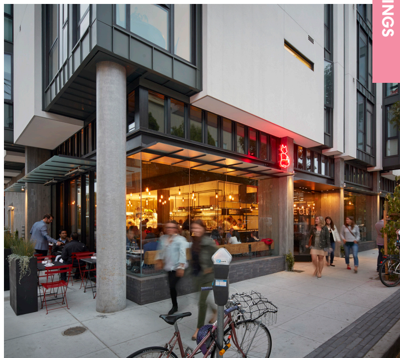
Figure 80 Ground floors can create notches of outdoor rooms to allow for lively spillover of retail.
