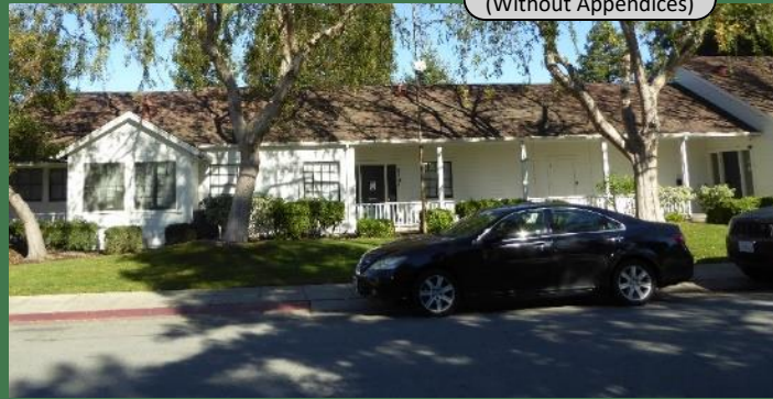
Figure 13 A portion of the southwest facade of the former office building. Source: Page & Turnbull
