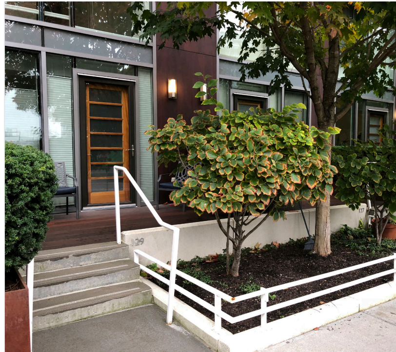
Figure 83 Ground floor residential stoops can provide privacy for residents and neighborhood beautification and Green Stormwater Infrastructure.
