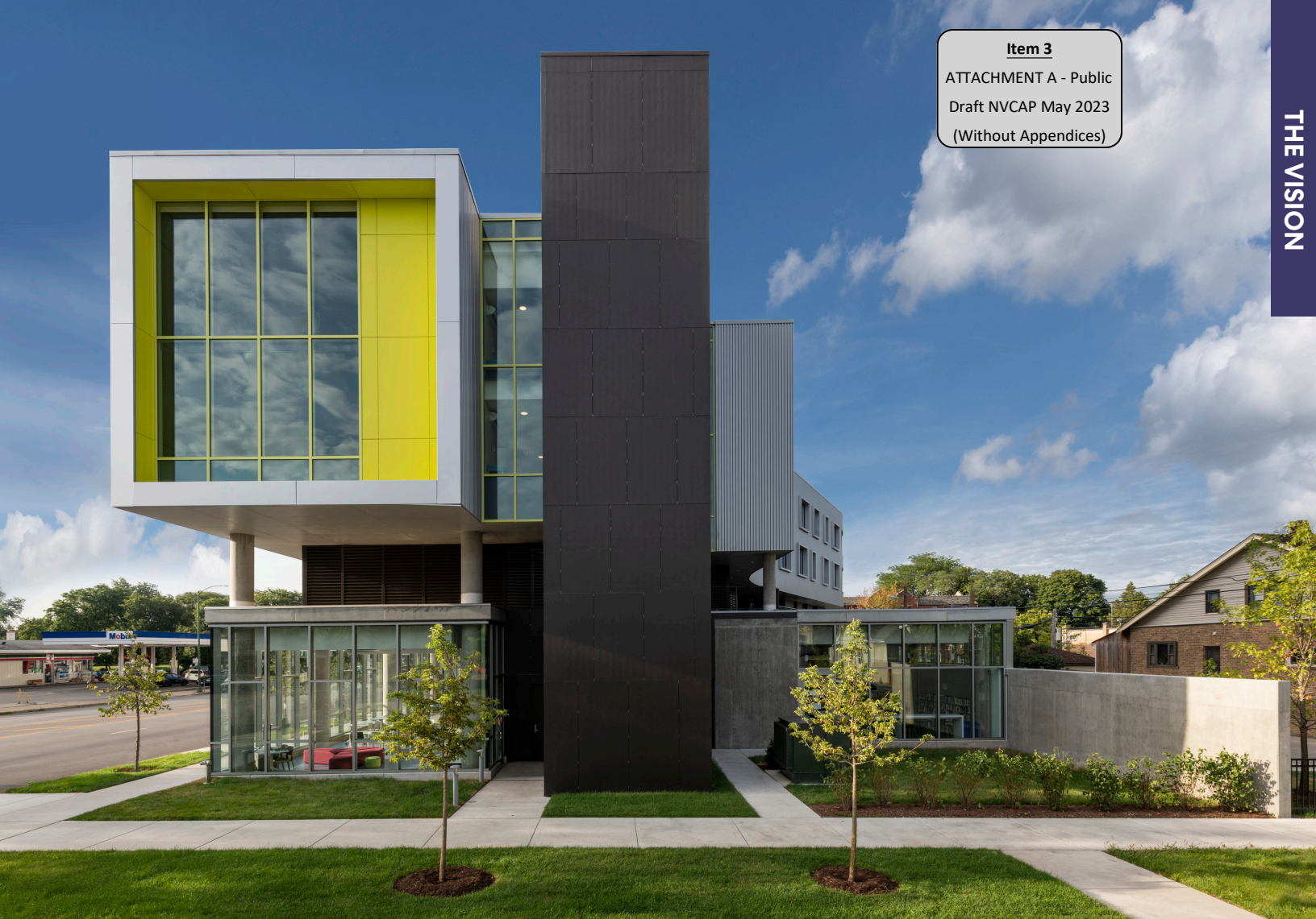
Figure 48 Urban form design standards requires setbacks and stepbacks for new development that is adjacent to single family zoning.
