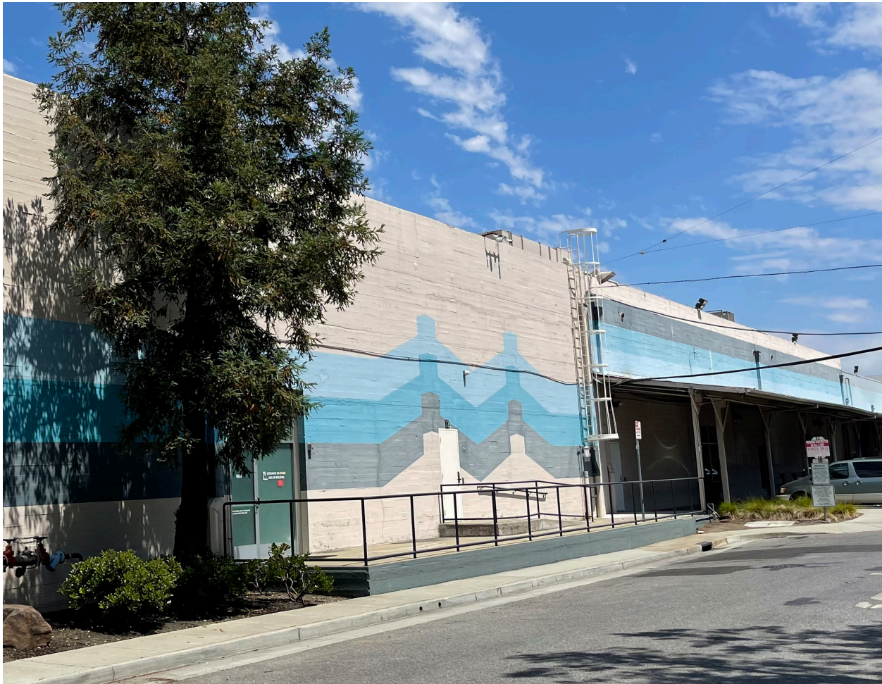
Figure 2 Photograph of the Cannery monitor roof supergraphic on the former Fry's site, 2022
