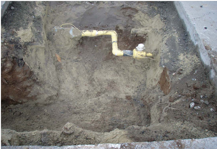
Installation of new HDPE gas service main
