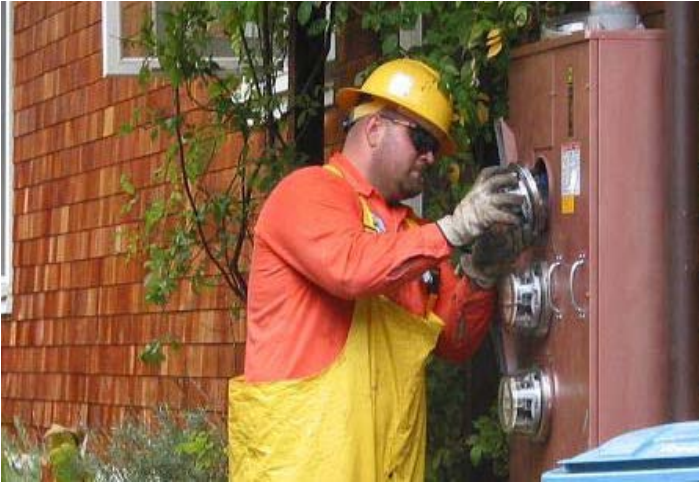
Electric Troublemaker installing an electric meter to provide service to a customer
