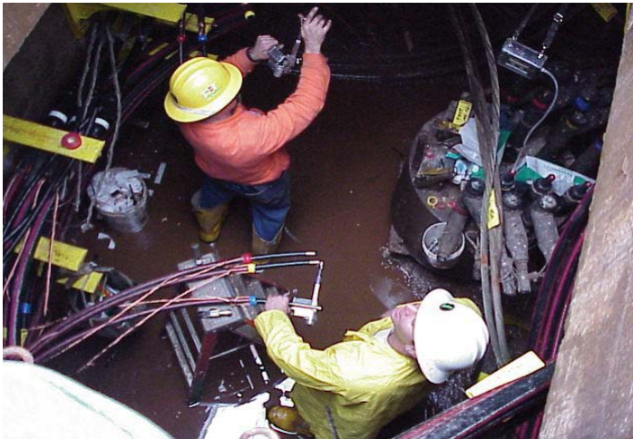
Electric crews working in an underground vault terminating cables
