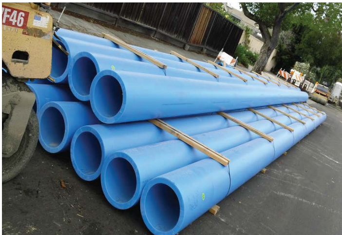
HDPE pipe waiting to be fused
