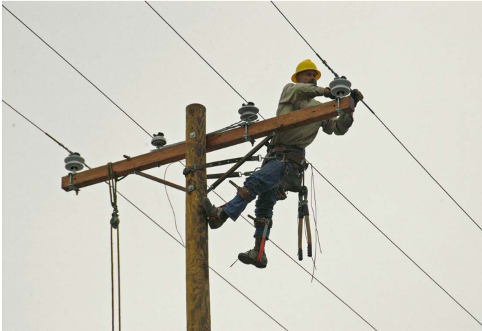
Electric Linemen working on utility pole
