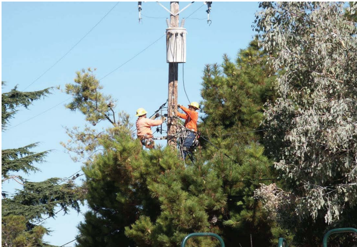
Overhead crews working on overhead lines
