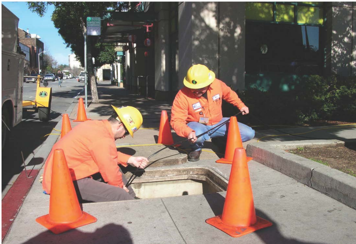
Fiber optic crew installing new fiber optic cables
