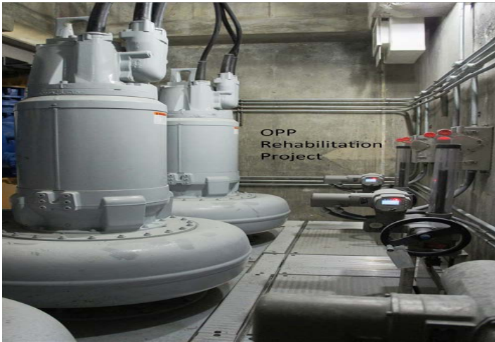
Old pumping plant
