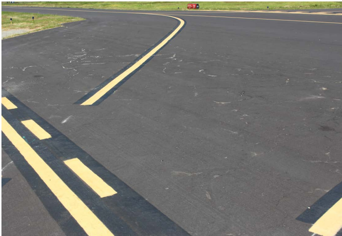
Runway and Taxiway, July 2017
