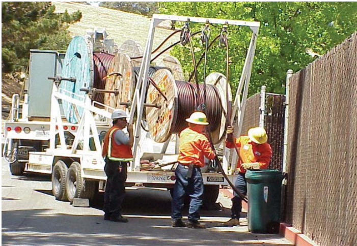
Electric crews installing new underground cables
