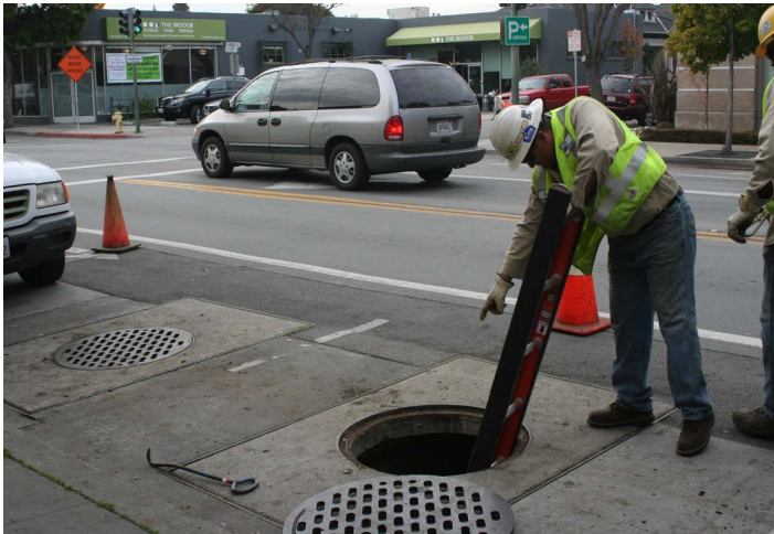
Electric crews preparing to enter underground vault
