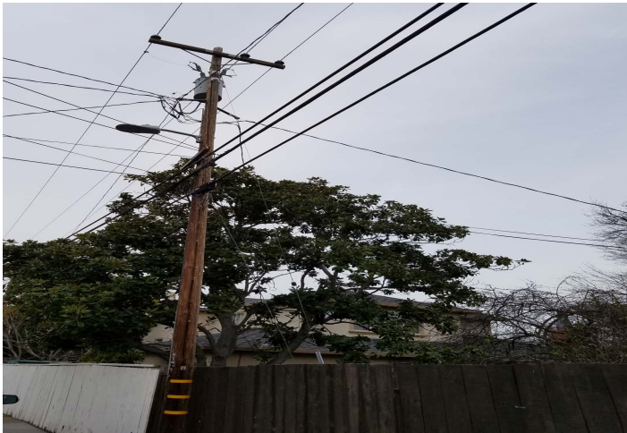
Aging pole that needs to be replaced.
