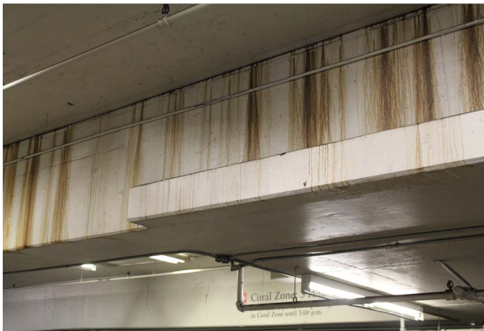
Civic Center Parking Garage, February 2015
