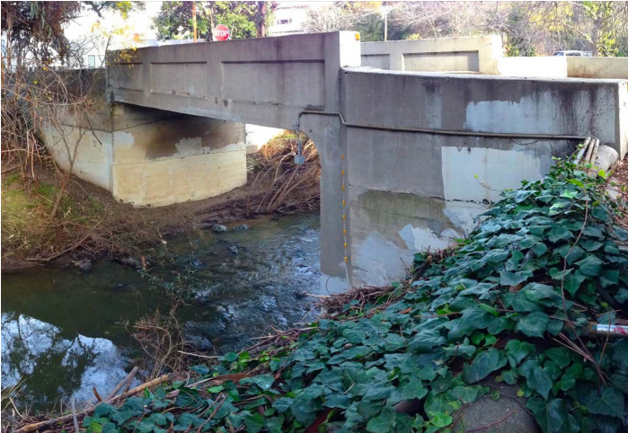
Newell Road Bridge, February 2015
