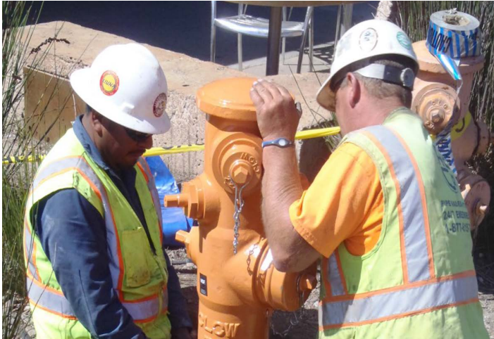
Installation of a new fire hydrant with FlowGuard fire hydrant check valve
