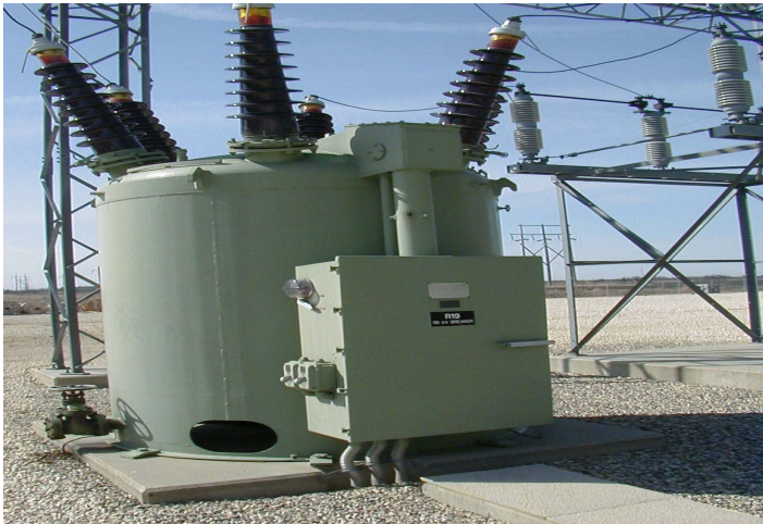
High voltage circuit breakers
