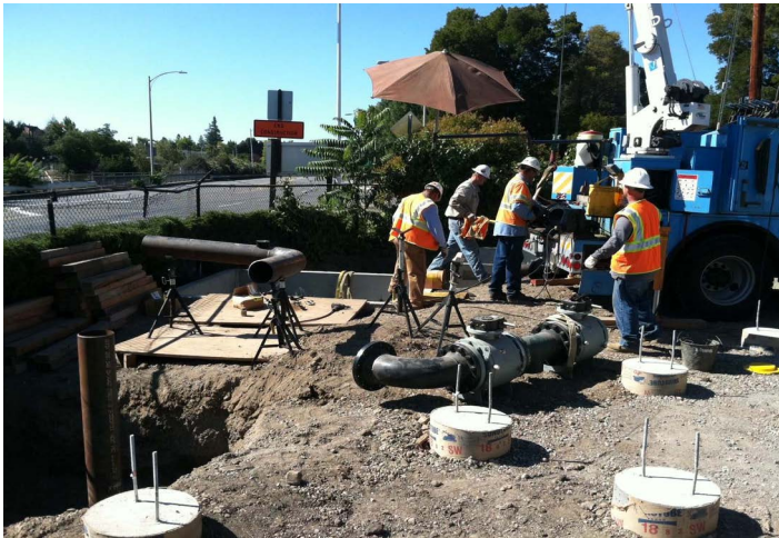
Installation of new HDPE gas service main
