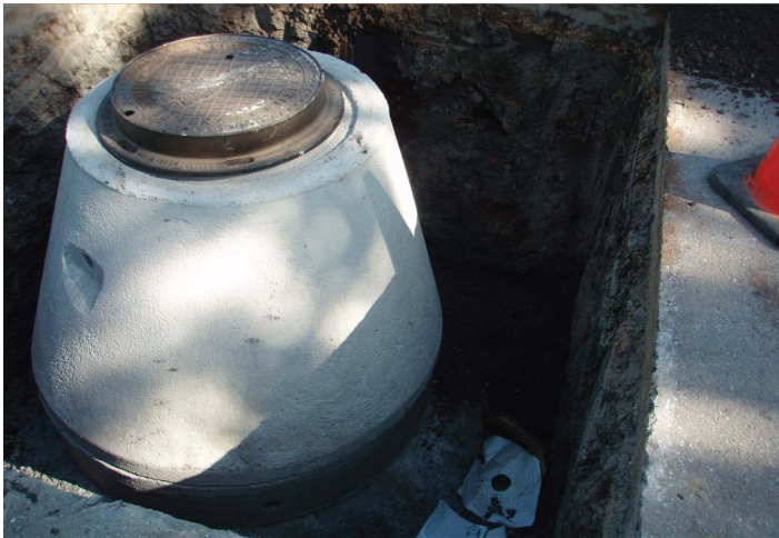
Sewer manhole base
