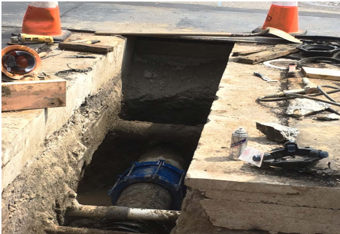
Installed 16" HDPE pipe waiting to be backfilled
