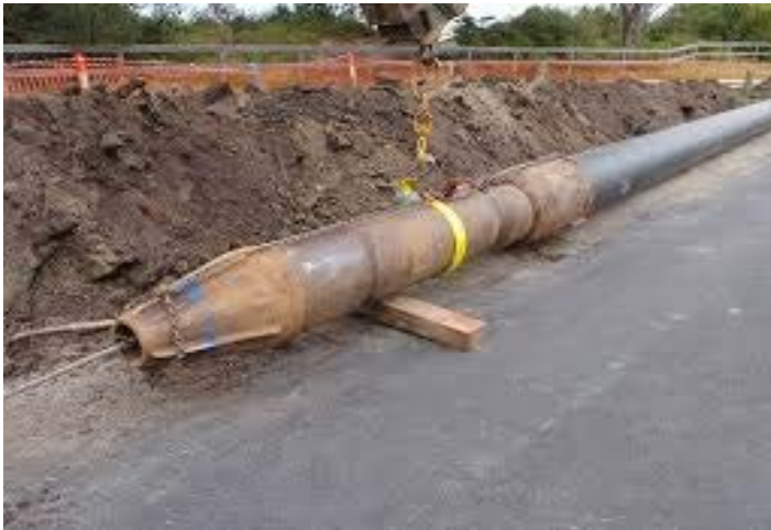
Sewer Main Replacement Project using Pipe Bursting Method
