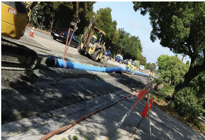
16" HDPE pipe ready to be installed by open trench method
