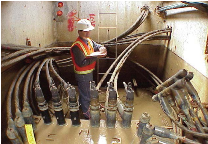
Utility Engineer planning out the next underground rebuild project
