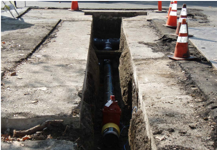
New HDPE main connecting to side street with new valve
