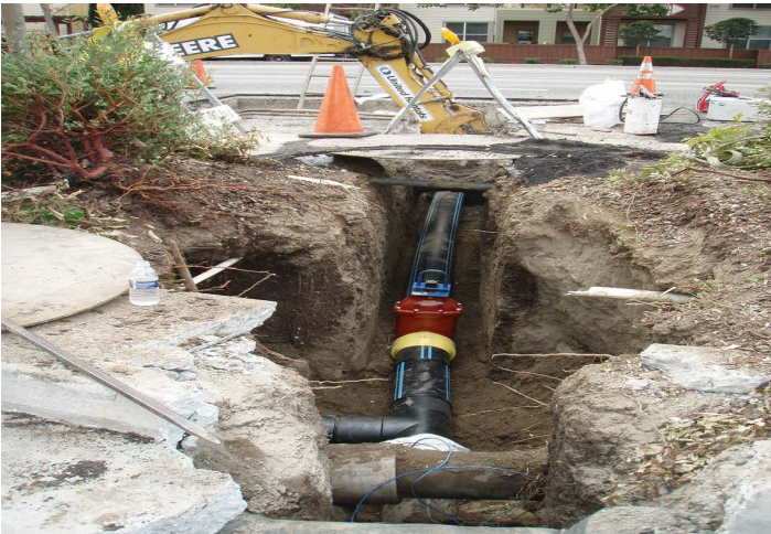
Installation of 8" HDPE pipe and valve between two main connection points on El Camino Real at El Camino Way
