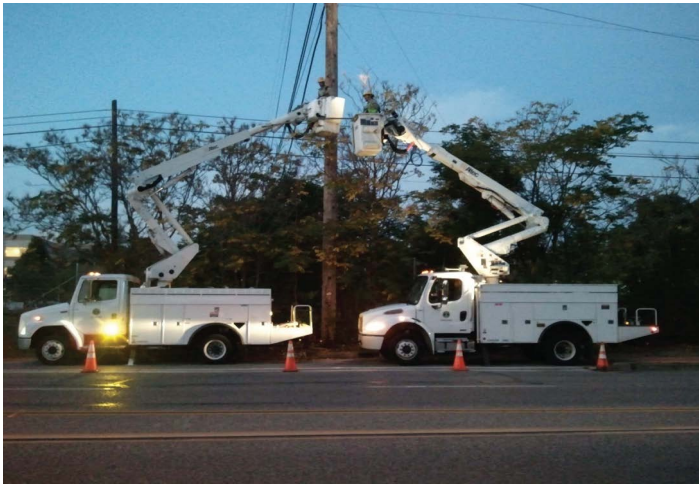
Traffic/Fiber technicians repairing the city fiber optic cables
