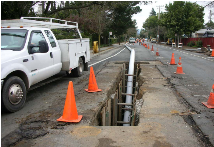
Sewer Trench Line
