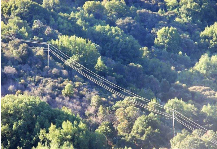
Overhead electric lines in Foothills Park
