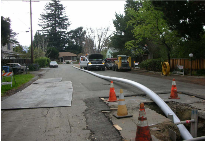
Trenching for installation of High Density Polyethylene (HDPE) sewer main by directional drilling method
