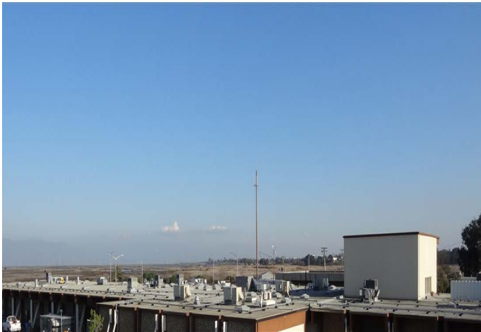
Municipal Services Center Building C, March 2015
