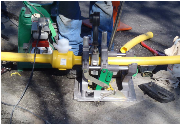
New HDPE gas pipe being fused prior to installation
