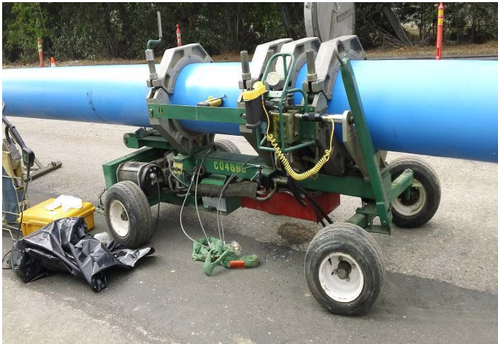
16" HDPE pipe being fused prior to installation
