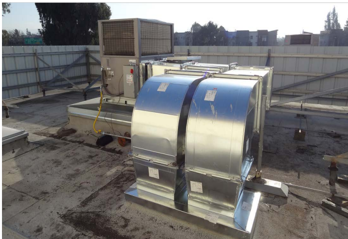
Municipal Service Center Building C Roof, January 2015
