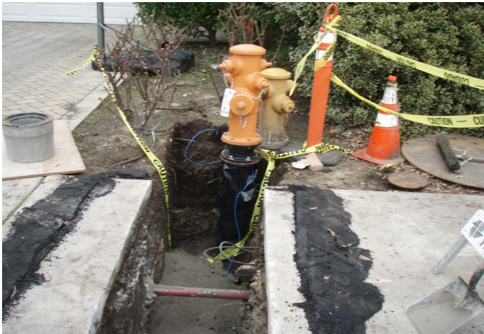
Newly installed fire hydrant service line and assembly on Greenwood Avenue
