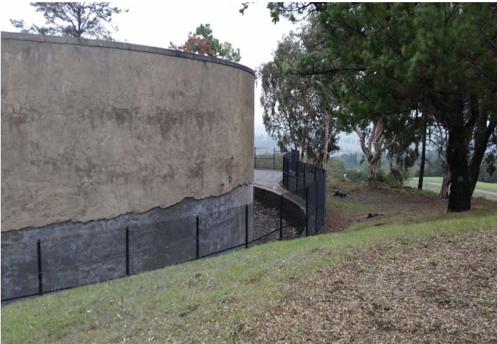
Seismic Upgrade, Boronda Reservoir, December 2014
