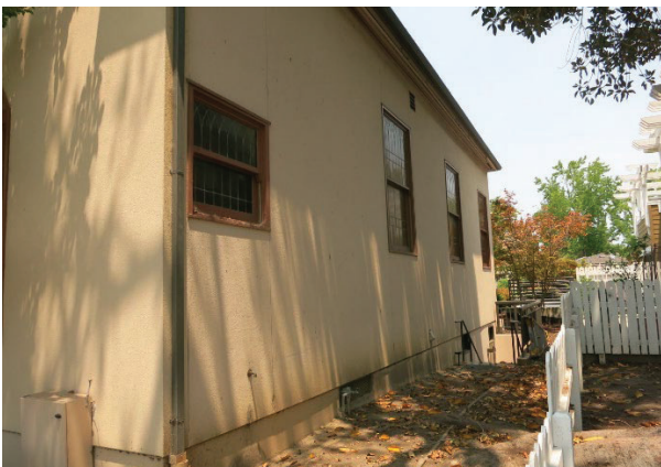
Figure 4: Detail of east façade. Looking northwest.
