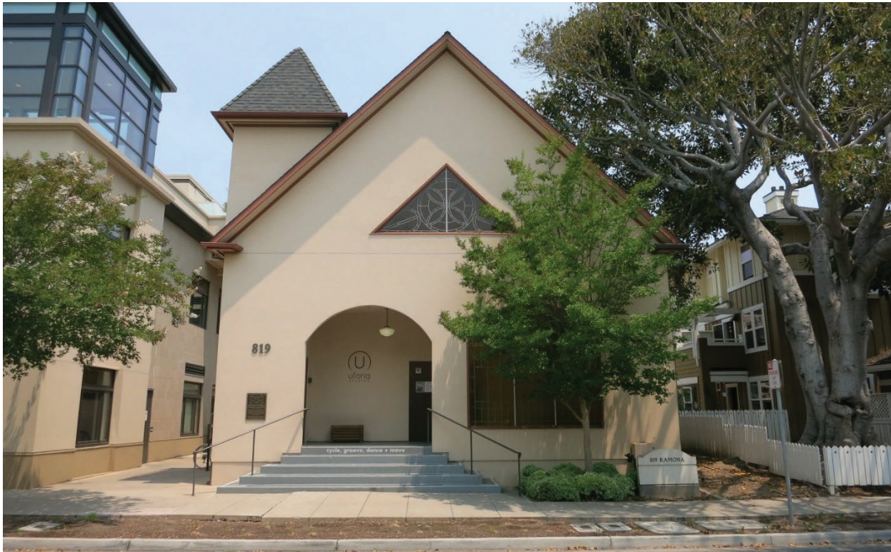
Figure 2: Primary (west) façade of the subject building. Looking east.
