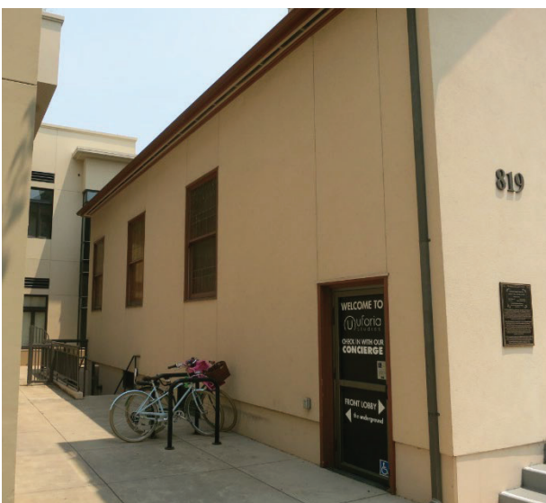
Figure 6: West façade, looking northeast.
