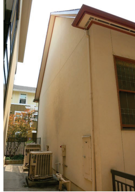
Figure 9: Rear (north) façade of the subject building. Looking southeast.
