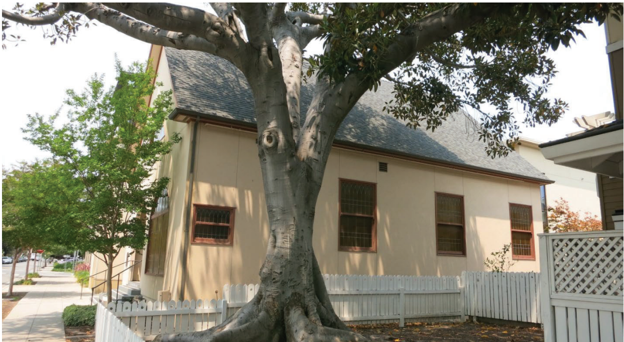
Figure 3: East façade of the subject building. Looking west.
