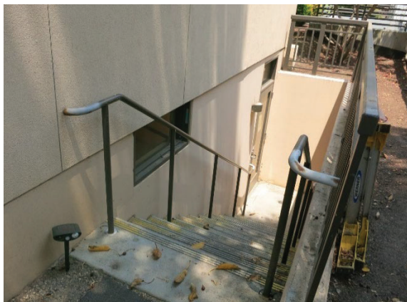
Figure 5: Detail of below-grade basement along east façade. Looking northwest.
