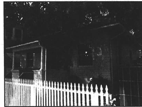
Figure 16. One-over-one, double-hung sash windows on Lytton Avenue facade (Photo: PAST Consultants).
