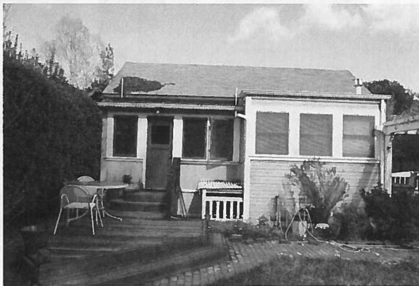
Figure 6: Rear (south) façade of 840 Kipling, looking north.
