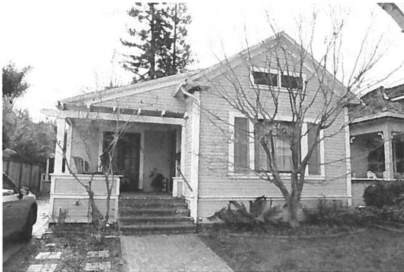
Figure 1: Primary (north) façade of 840 Kipling, looking south.
