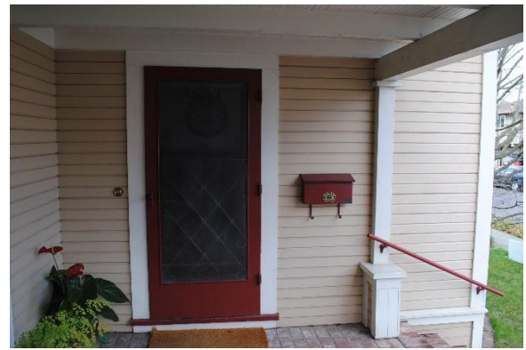
Figure 3: Primary entrance door on the east-facing wall of the front porch.
