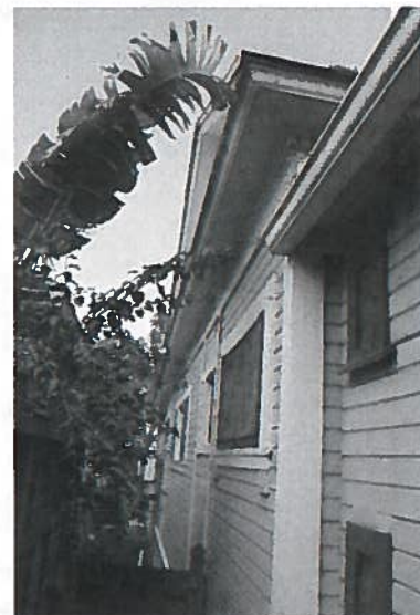
Figure 10: Partial view of west façade, facing north.
