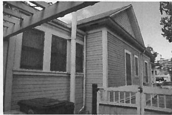
Figure 5: Partial view of east façade, facing north. Flat-roof volume visible at the left is located at the rear of the residence.
