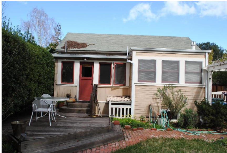
Figure 6: Rear (south) façade of 840 Kipling, looking north.
