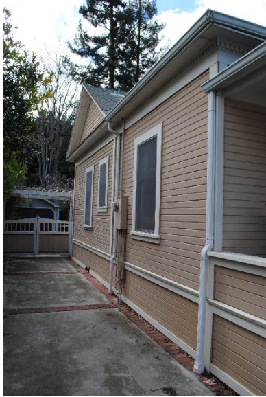
Figure 4: Partial view of east façade, facing west.
