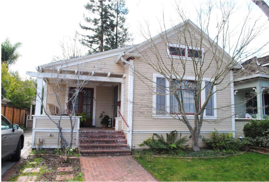
Figure 1: Primary (north) façade of 840 Kipling, looking south.
