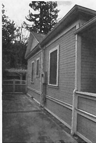
Figure 4: Partial view of east façade, facing west.
