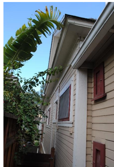
Figure 10: Partial view of west façade, facing north.
