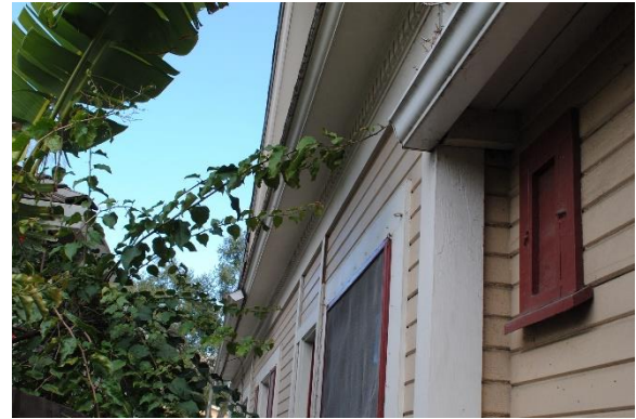
Figure 8: Connection between the flat-roofed rear volume and main volume of the residence, looking north along the west façade. The siding is not aligned, and the roof eave detailing differs from the main volume.
