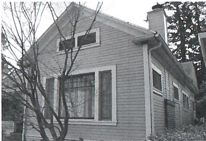
Figure 9: Partial view of west façade (right), looking south.
