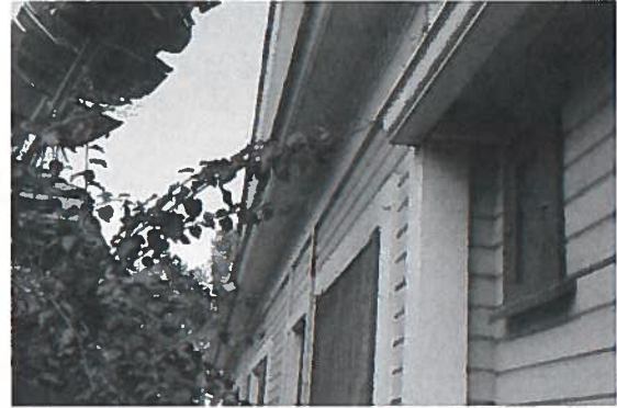
Figure 8: Connection between the flat-roofed rear volume and main volume of the residence, looking north along the west façade. The siding is not aligned, and the roof eave detailing differs from the main volume.
