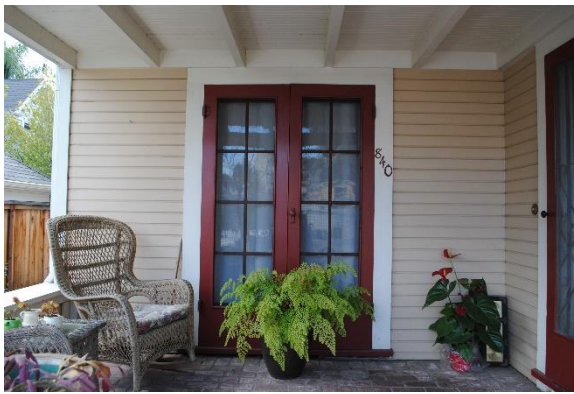
Figure 2: Fully-glazed double doors on north-facing wall of the front porch.
