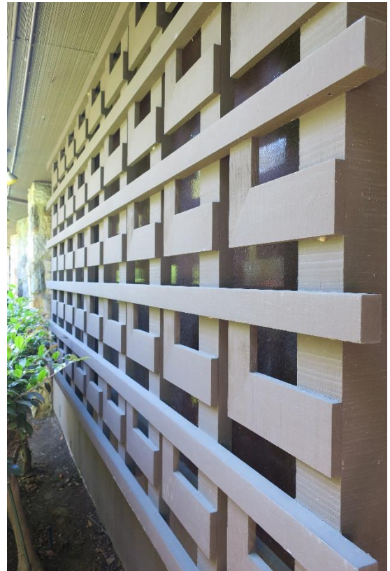
Figure 13: Geometric wood screen shielding opaque fixed window, view looking southeast.
