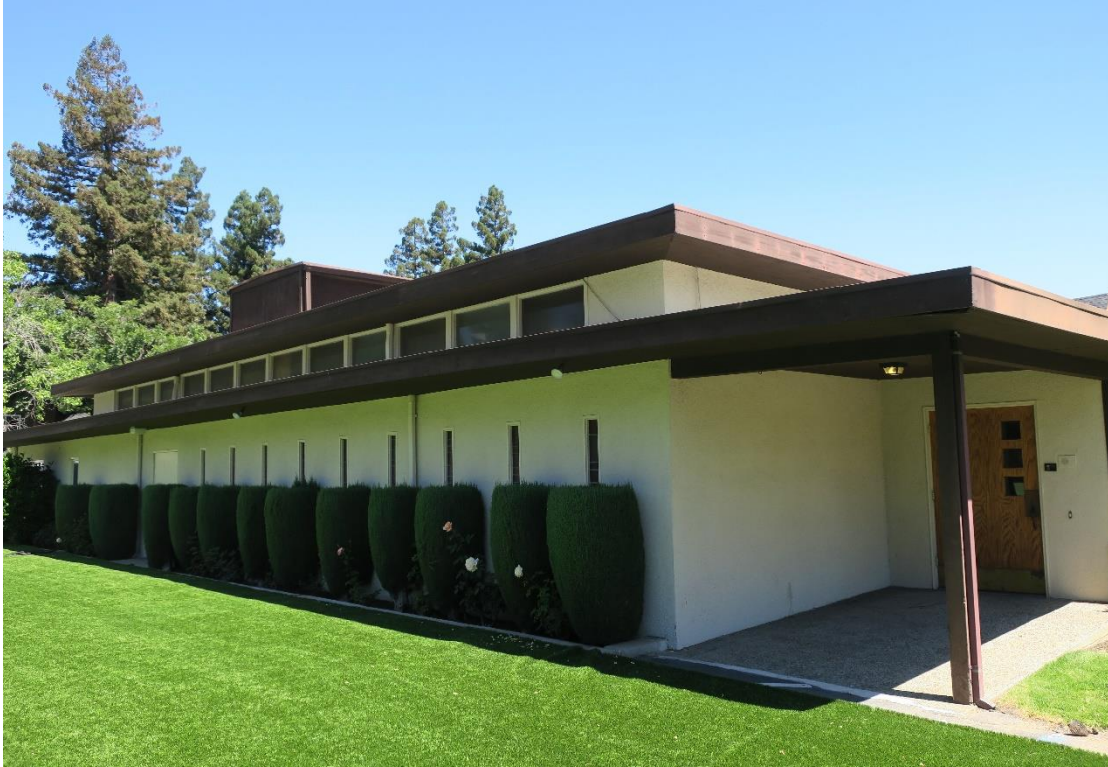
Figure 23: Central portion of southwest façade, view looking northwest.
