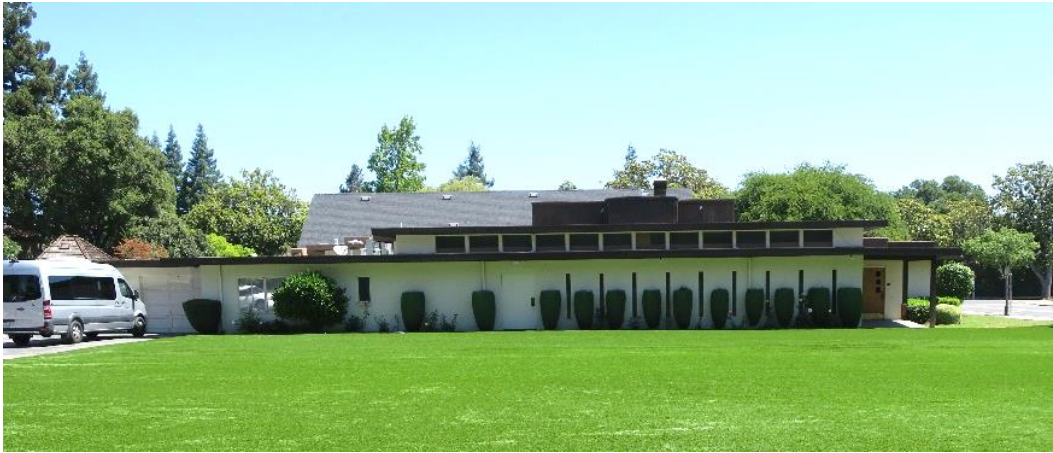
Figure 18: Rear southwest façade, view looking northeast.
