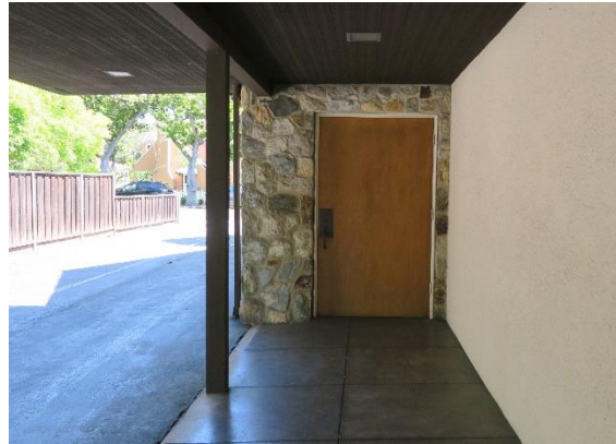
Figure 15. Stone wall and wood door leading into double-height volume, view looking northeast.
