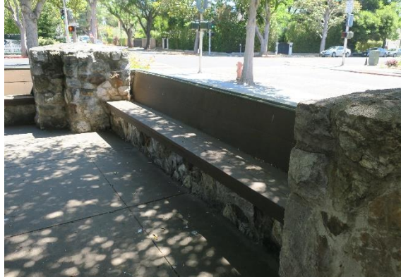
Figure 30: Partial-height stone wall with wood bench, view looking east.
