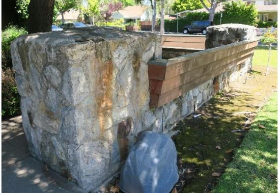
Figure 29: Partial-height stone wall with wood bench, view looking north.
