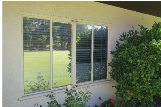
Figure 20: Two casement windows with outer fixed lites, view looking east.
