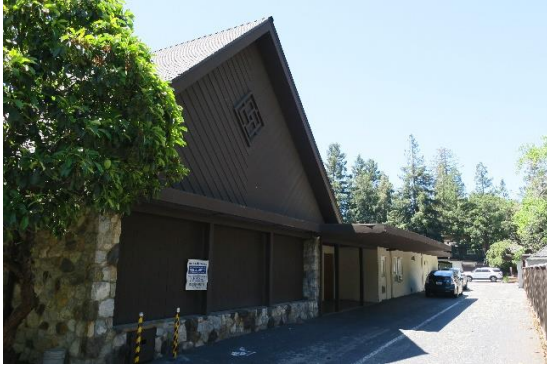
Figure 35: Driveway at northwest façade, view looking southwest.
