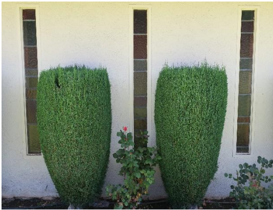
Figure 24: Detail of stained glass vertical ribbon windows.
