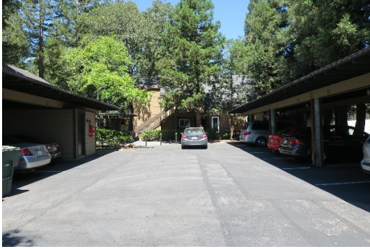
Figure 42: Webster Wood Apartments.
