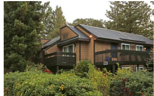
Figure 45: Webster Wood Apartments. Source: Apartments.com
