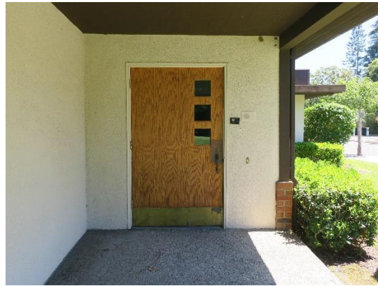
Figure 25: Recessed vestibule at the far right (south) portion of the southwest façade, view looking northeast.
