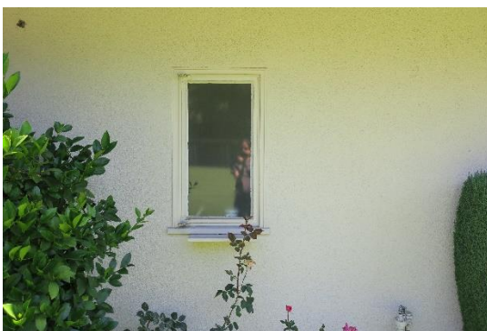
Figure 21: Single casement window, view looking northeast.
