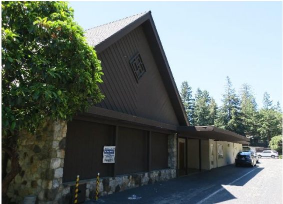
Figure 14. Northwest façade, view looking south.
