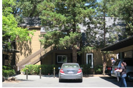
Figure 43: Webster Wood Apartments.
