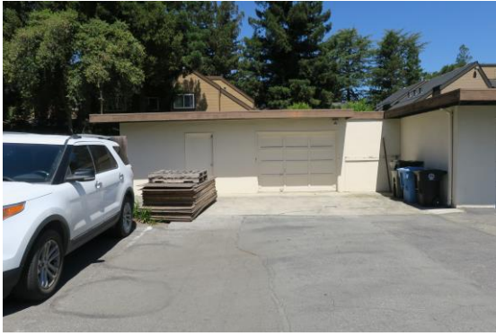
Figure 40: Garage, view looking northwest.
