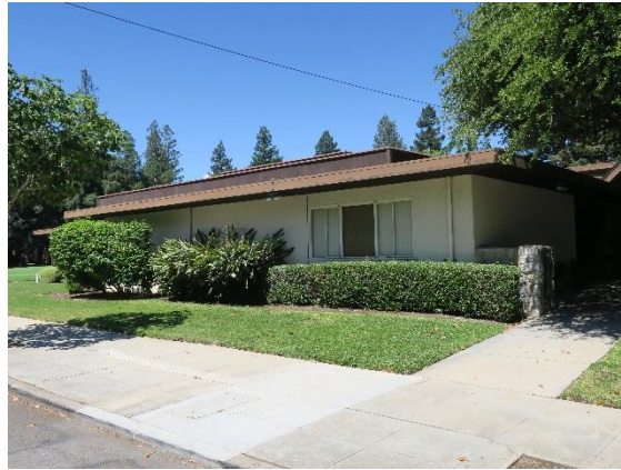
Figure 28: Southeast façade, view looking west.
