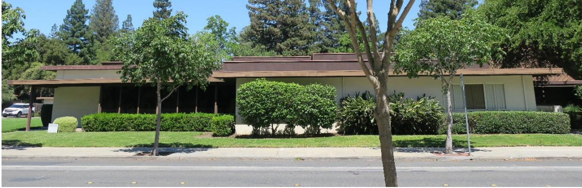
Figure 26: Southeast façade, view looking northwest.
