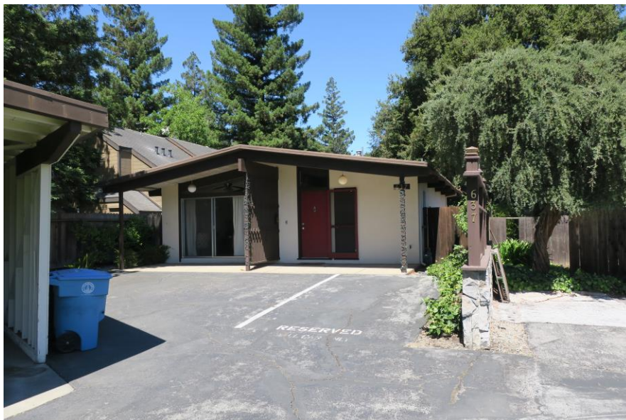
Figure 39: One-story caretaker residence at 637-45 Addison Avenue (built 1964).
