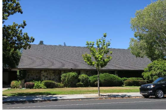
Figure 11: Main sawtooth portion of primary façade fronting Middlefield Avenue, view looking southwest.
