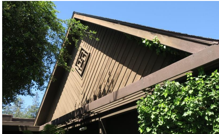
Figure 9: V-pattern wood siding within southeast-facing open gable, with central geometric relief.
