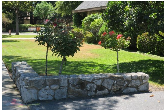
Figure 34: Partial-height stone wall, view looking southeast.
