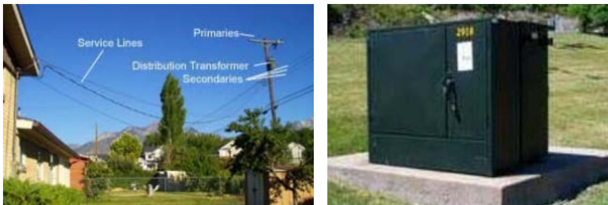
Figure A.3: Pole-top Vs Pad-mounted Distribution Transformers
