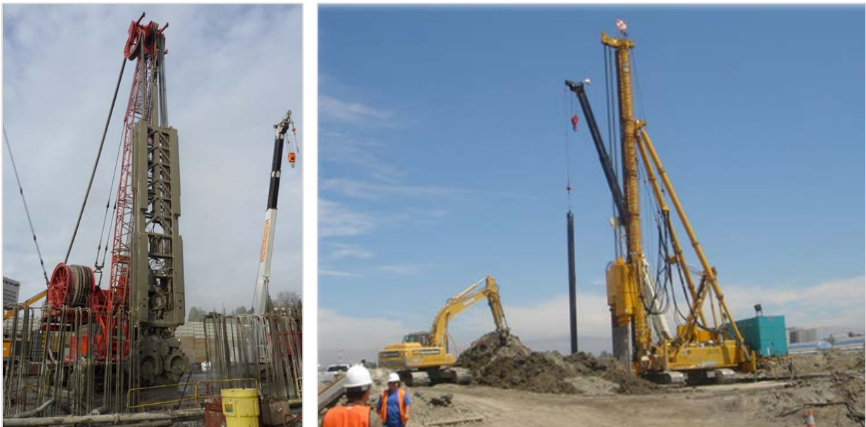
Figure 8: Typical Support of Excavation (SOE) Wall Installation Equipment
