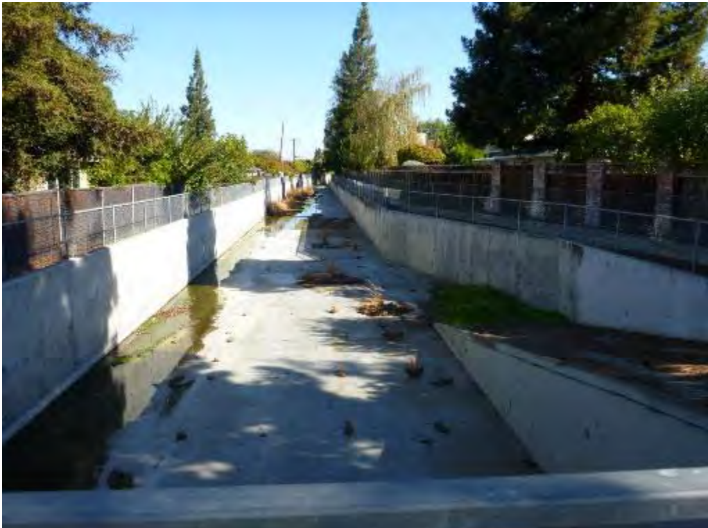
Photo 5: Adobe Creek crossing along Middlefield Road, facing northwest.
