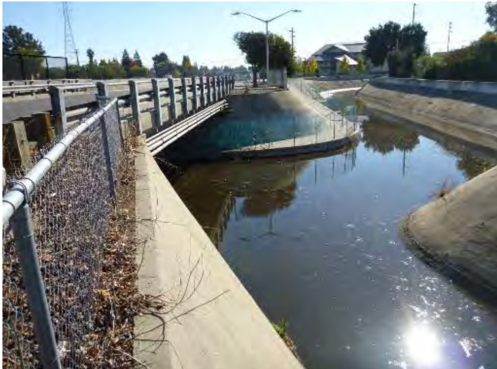
Photo 3: Adobe Creek crossing along West Bayshore Road, facing southeast.
