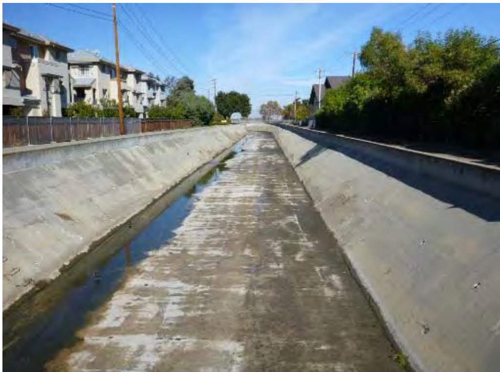
Photo 4: Adobe Creek crossing along East Meadow Drive, facing north.
