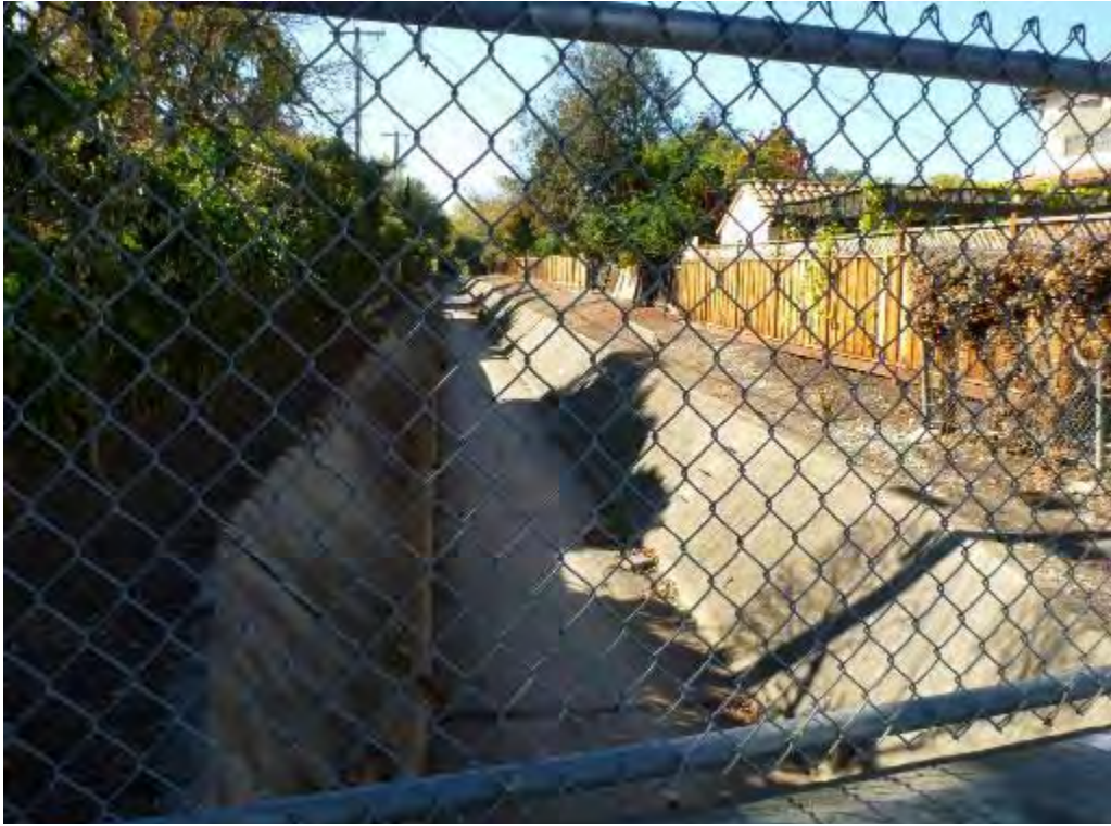
Photo 7: Barron Creek crossing along Cowper Street, facing southwest.
