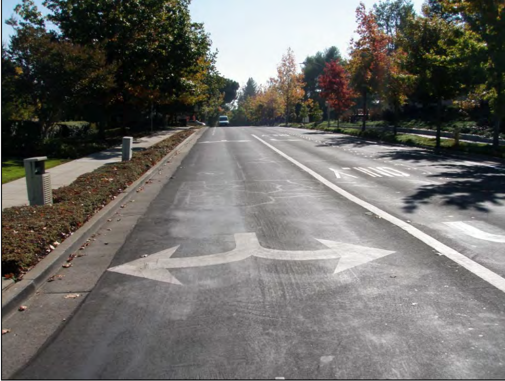
Photo 9: View E along Porter Drive from Page Mill Rd.
