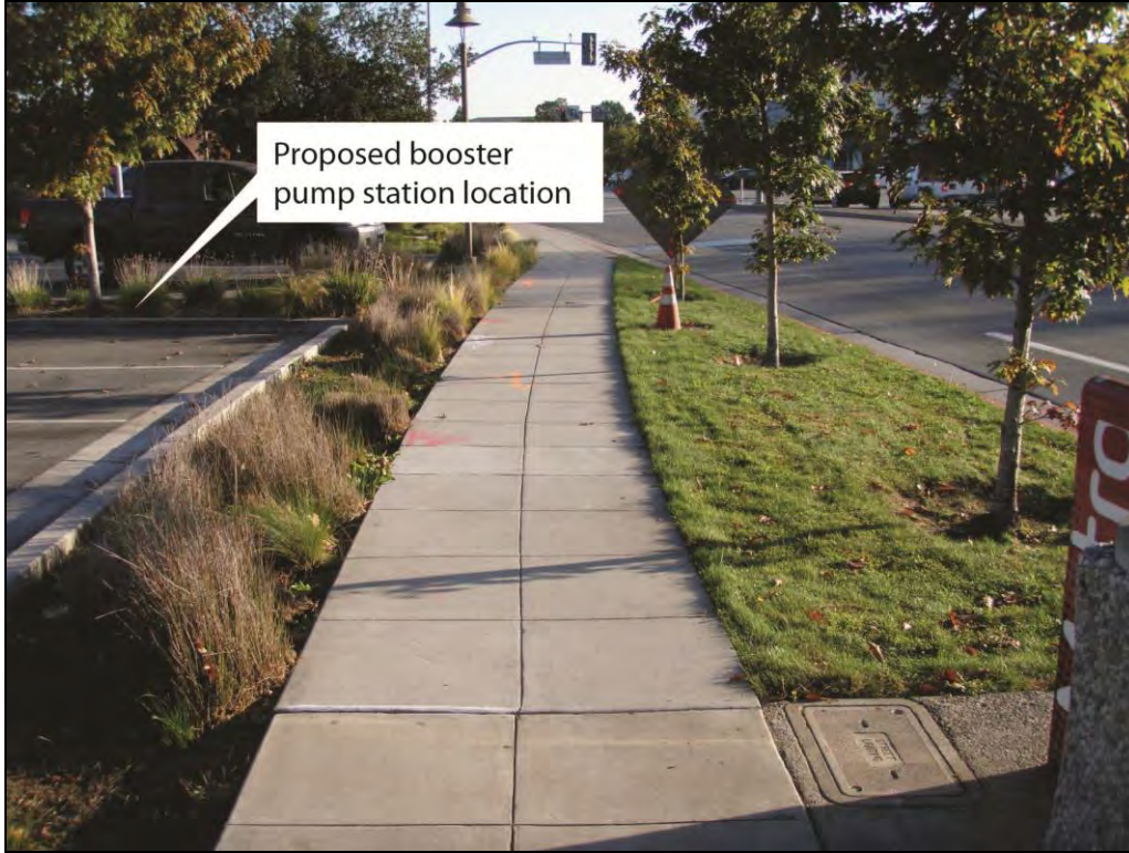
Photo 17: View NE along Page Mill Rd. -- proposed booster pump station location (arrow).
