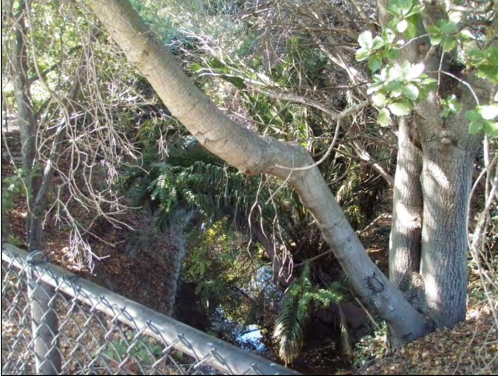
Photo 5: View NE along Matadero Creek at the Hillview Ave. crossing.
