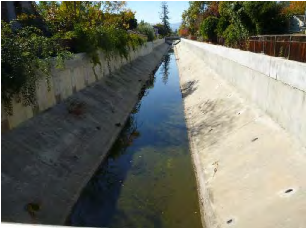
Photo 8: Matadero Creek crossing along Cowper Street, facing southwest.
