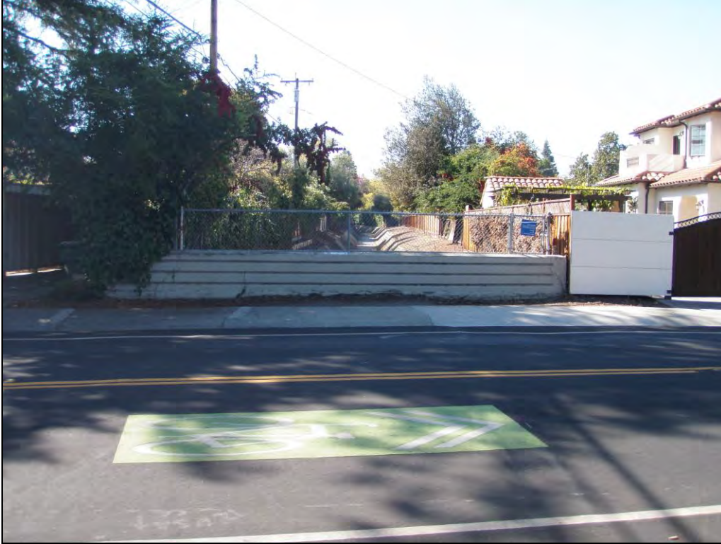
Photo 3: View SW along Barron Creek at the Cowper Street crossing.
