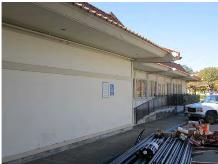
Figure 8 East Elevation. Photo taken Nov 12, 2015
