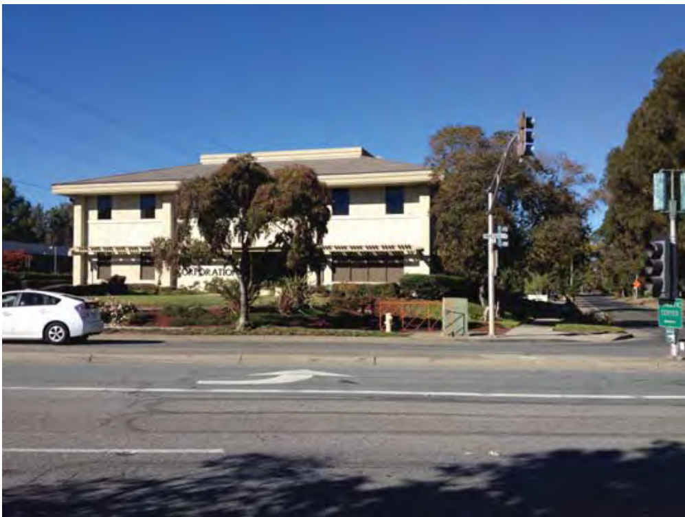
Photo 2: Office building across Embarcadero Road north of project site
