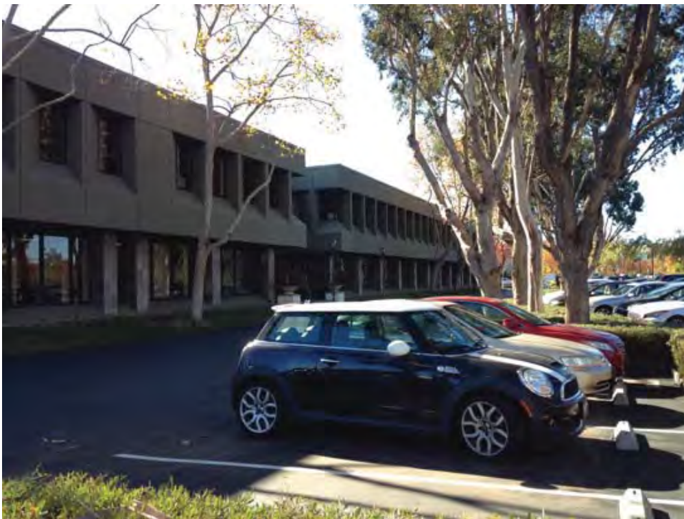
Photo 2: Office building south of project site
