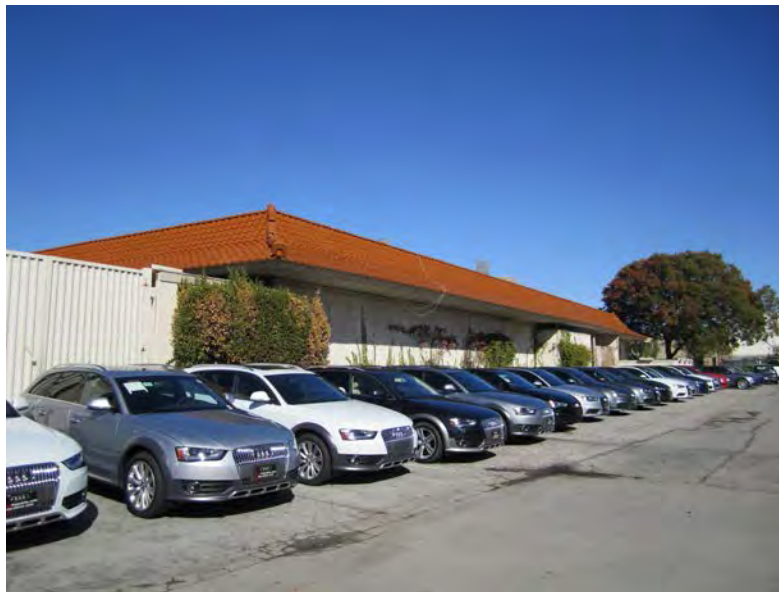
Figure 6 South (Rear) elevation. Photo Taken Nov 12, 2015
