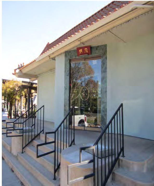
Figure 1 Front (North) Entrance Facing Embarcadero Road. Photo taken Nov 12, 2015.
