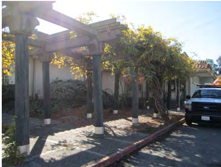
Figure 2 Path to Former Entry at northeast corner. Photo taken Nov 12, 2015
