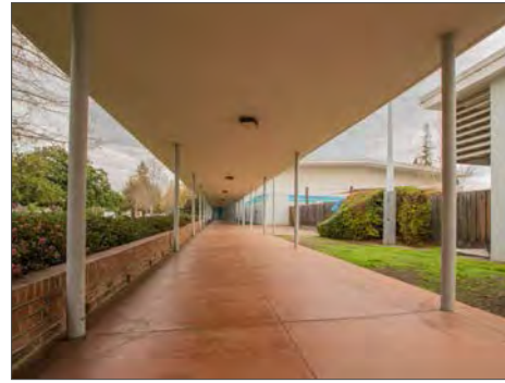
A | Outdoor covered walkways
