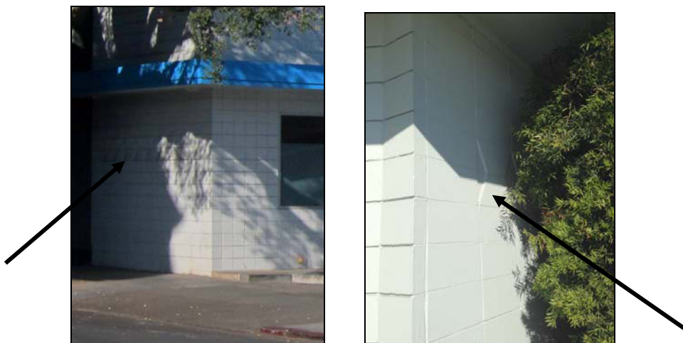
Figures 3 and 4. Decorative concrete blocks on Emerson Street, left; and Forest Ave, right (arrows).
