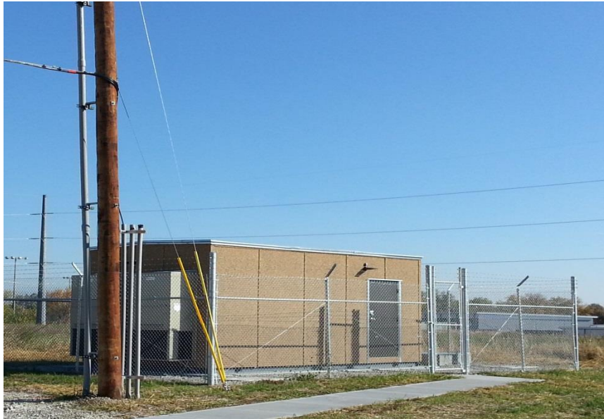
Fiber Network Hut
