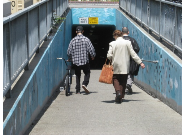
The California Avenue undercrossing is frequently used, but it is narrow and challenging for pedestrians with disabilities.
