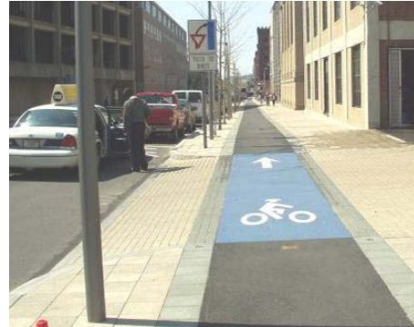
Colored pavement informs bicyclists and drivers of a potential conflict area.
