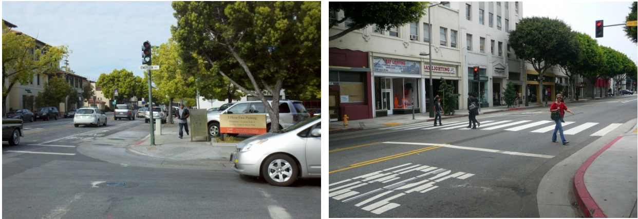
A typical signalized crossing in Palo Alto (left) compared to a best practice crossing treatment (right). Differences include a higher visibility “continental” striping pattern and “advance stop bar” to limit encroachment by vehicles; pedestrian countdown signals; curb extensions or “bulb outs” to reduce crossing distances and vehicle turn speeds; and curb ramps with color contrasting detectable warning strips. For more detail on specific pedestrian crossing treatments, see Appendix A.A
