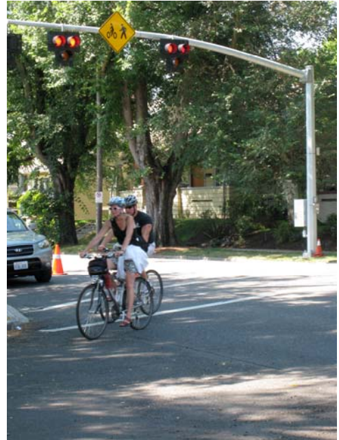
HAWK signal in Portland, OR assists with an arterial crossing on a bicycle boulevard. Note the use of the combined pedestrian/bicycle warning sign (W11-15).
