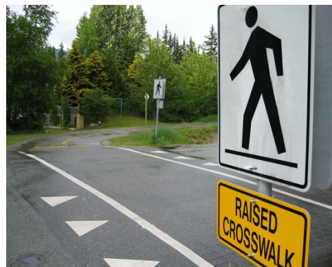
Raised crosswalks calm traffic while enhancing pedestrian crossings.
