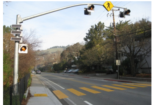
An overhead solar-powered beacon assists a crossing of Sir Francis Drake in San Anselmo, CA.
