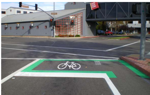
San Luis Obispo uses a simpler version of a bike box. Source: Caltrans.
