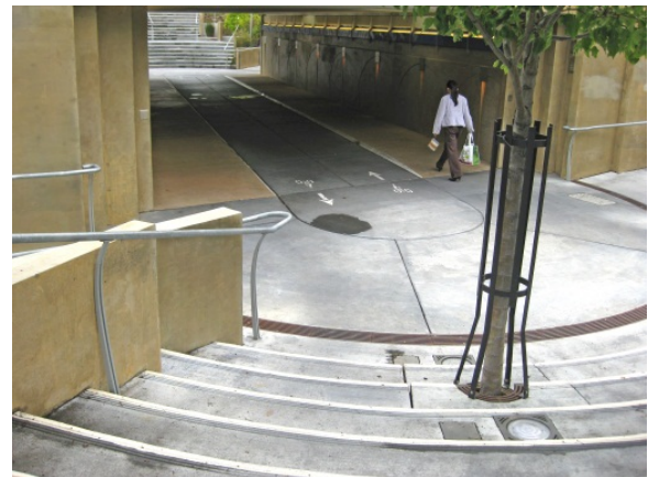
The Homer Street Underpass is the most recent barrier crossing improvement in the City of Palo Alto and accommodates both pedestrians and bicyclists.
