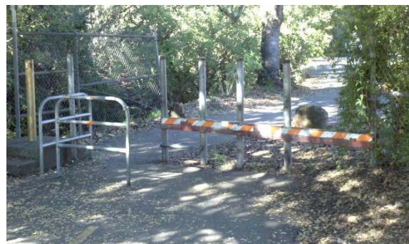
Gunn High School Path at the terminus of Los Robles Avenue. This barrier design is typical of many existing trail intersections, and complicates use by people with disabilities, strollers, and bicycles with trailers.
