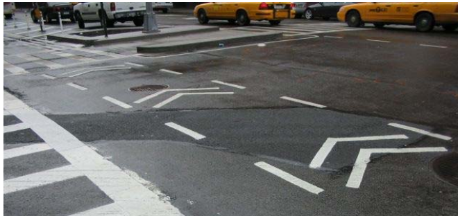
Dashed lines and chevrons delineate bicyclist path of travel through an intersection on the 9 th Avenue cycletrack in New York City.
