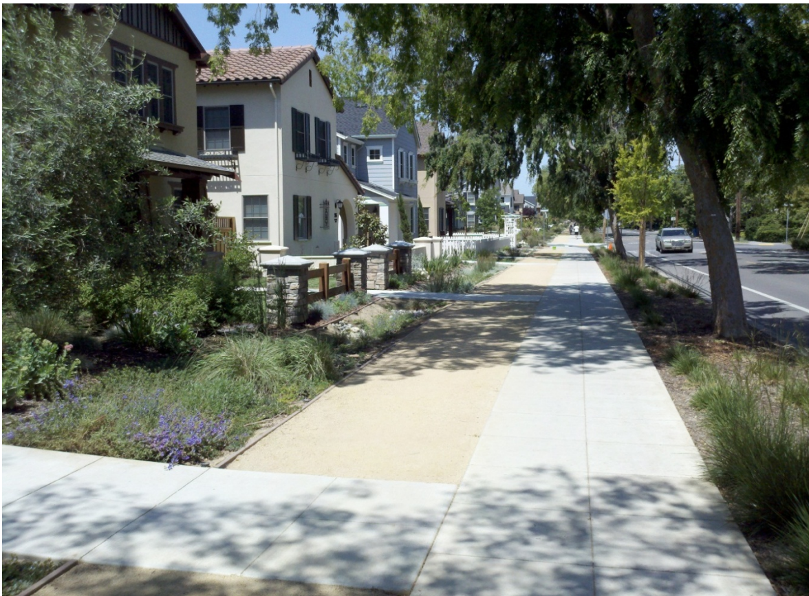
The new sidewalk constructed along Stanford Avenue adjacent to a faculty housing development includes both a paved and unpaved surface to support utilitarian and recreational (jogging) pedestrian activity. This hybrid walkway extends from Hanover Street to El Camino Real along the Bay to Ridge Trail.
