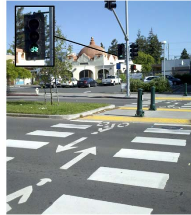
A bicycle signal is paired with a wider crosswalk to accommodate bicyclists in Berkeley, CA to assist with the Ohlone Greenway crossing of University Avenue.
