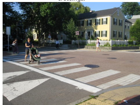
Raised intersections also calm traffic, but can be expensive due to drainage issues.
