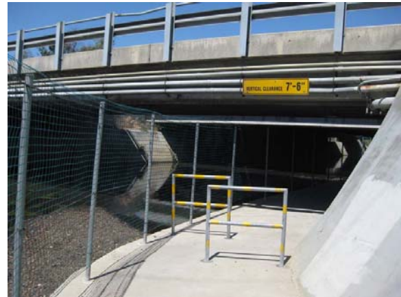
Despite being open only five months out of the year due to seasonal flooding, the Adobe Creek Underpass carries an estimated 43,000 annual users.
