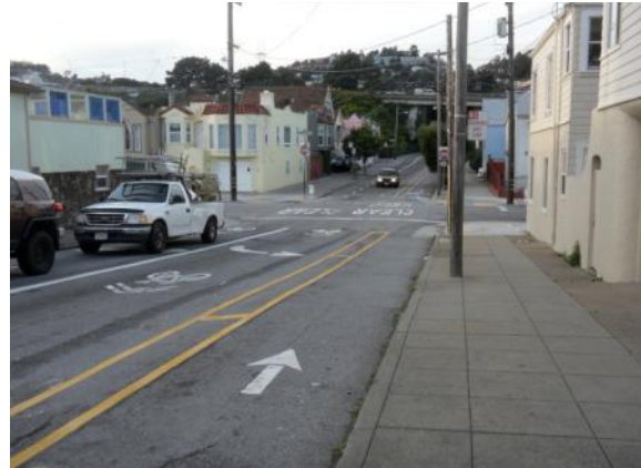
The City of San Francisco installed a contra flow bike lane on Lyell St. Photo Credit: Eric Fischer
