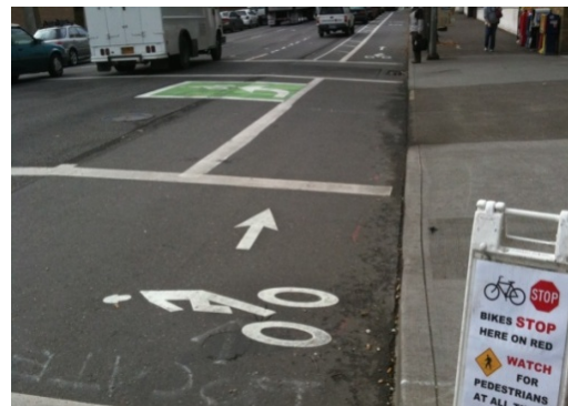
Bike box positions bicyclists to make a left turn from a cycle track in Portland, OR.
