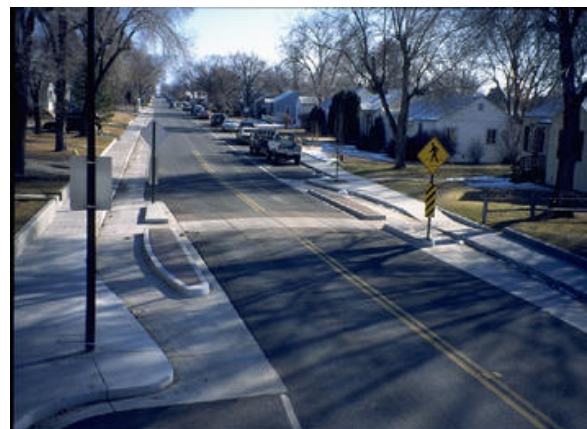
This choker shortens a mid-block crosswalk and provides a channel for bicyclists and drainage.
