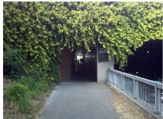
The University Avenue/Palo Alto Transit Center undercrossing is narrow and has poor visibility.
