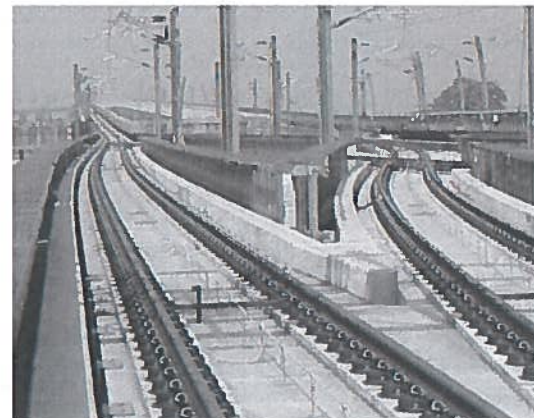
Figure 10 Photo of KCRC viaduct completed
