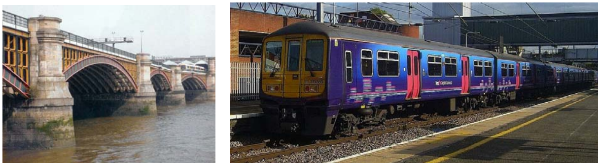
Figure 34: Left: View of Blackfriars Railway Bridge from the south bank. Right: First Capital Connect Class 319 EMU.
