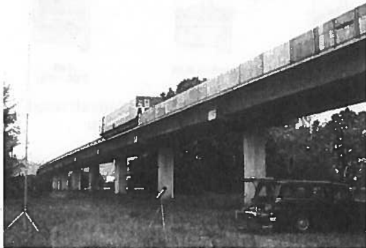
Figure 2 Photo of BART Test Track concrete viaduct and trial sound barrier wall
