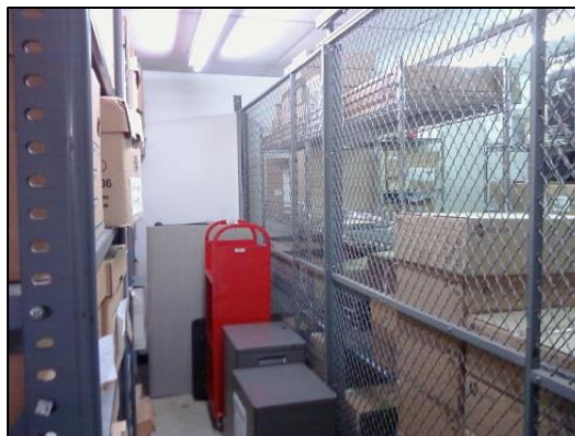
Exhibit 19: Inadequate fencing allows access to IT assets
