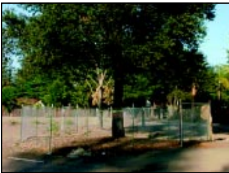
IMAGE 2.15-2 Tree Protection Fence at the Dripline
