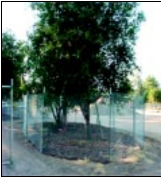
IMAGE 2.15-1 Tree Protection Fence at the Dripline
