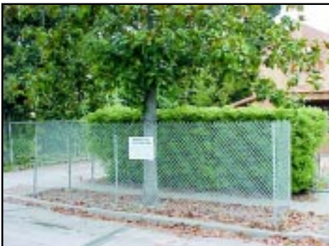
IMAGE 2.15-3 Tree Protection within a Planter Strip
