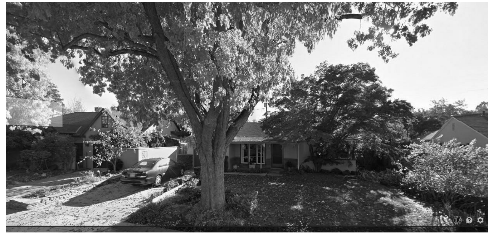
# 4118 ( PROJECT SITE) EXISTING BLDG. TO BE REMOVED
