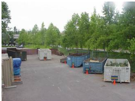
Construction materials are collected on-site for recycling
