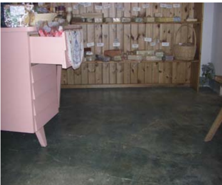
Soy based stain was used to color the concrete floor
