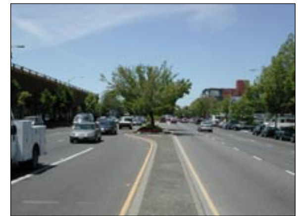
Figure 2.3: Narrow median on El Camino today.
