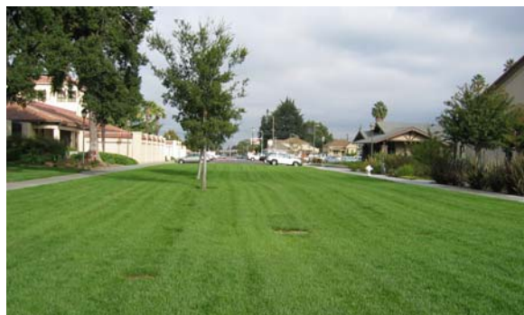
Turf block fire access road, Santa Clara
